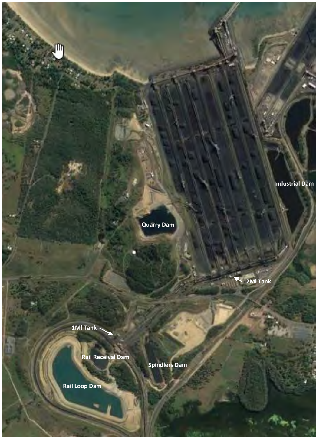
Figure 7: Water Management Infrastructure
