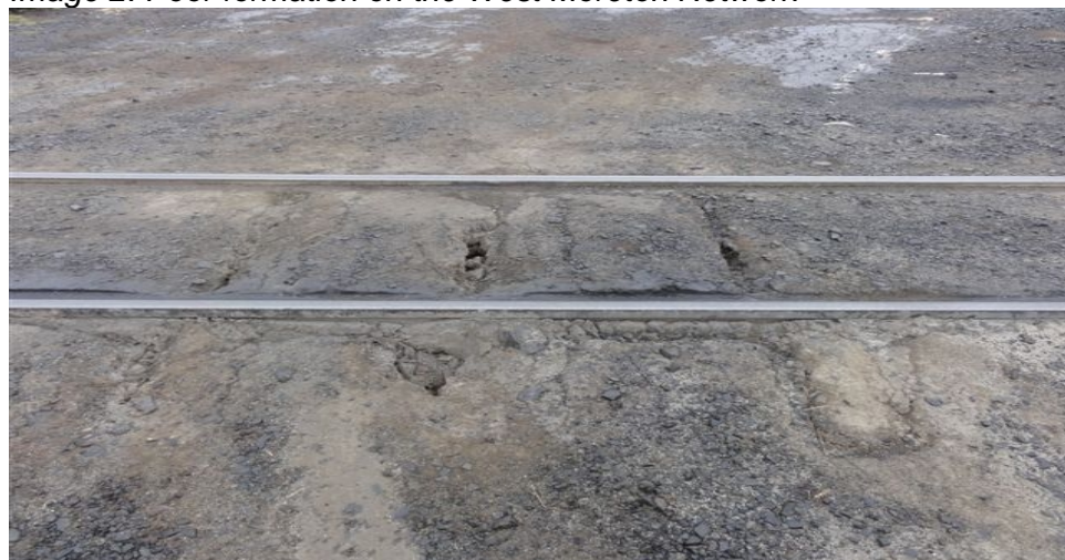
Image 2: Poor formation on the West Moreton Network
