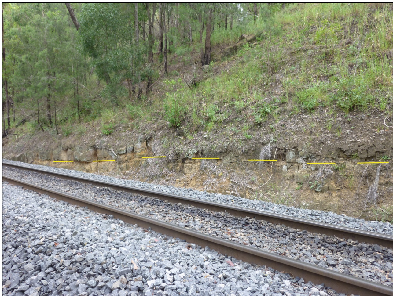
Photograph 3: View north from Borehole BH01 at approximate Ch 144.8 km showing in situ extremely weathered rock exposed in the upslope cutting adjacent to the rail line (sandstone above and mudstone below the yellow dashed line).
