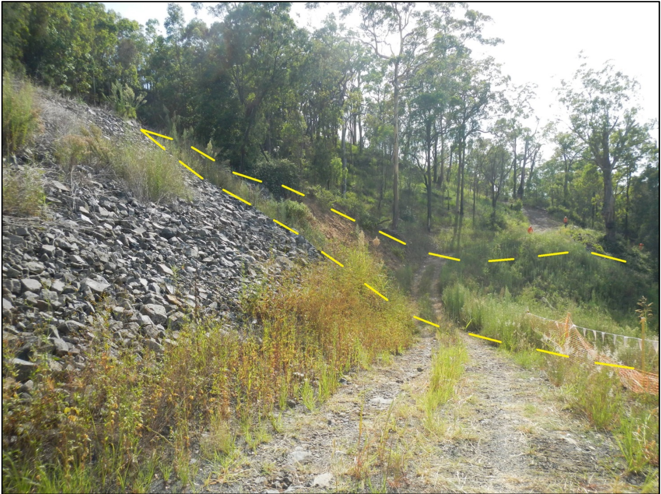
Photograph 8: View east along the lower access road from Borehole BH06 showing the location of the landslide centred on approximate Ch 144.55 km (yellow dashed lines). Note: some minor remedial works have been undertaken by QR to re-instate the lower access road within the landslide zone, however the slopes immediately above and below the road remain untouched since the time of the failure in February 2013.
