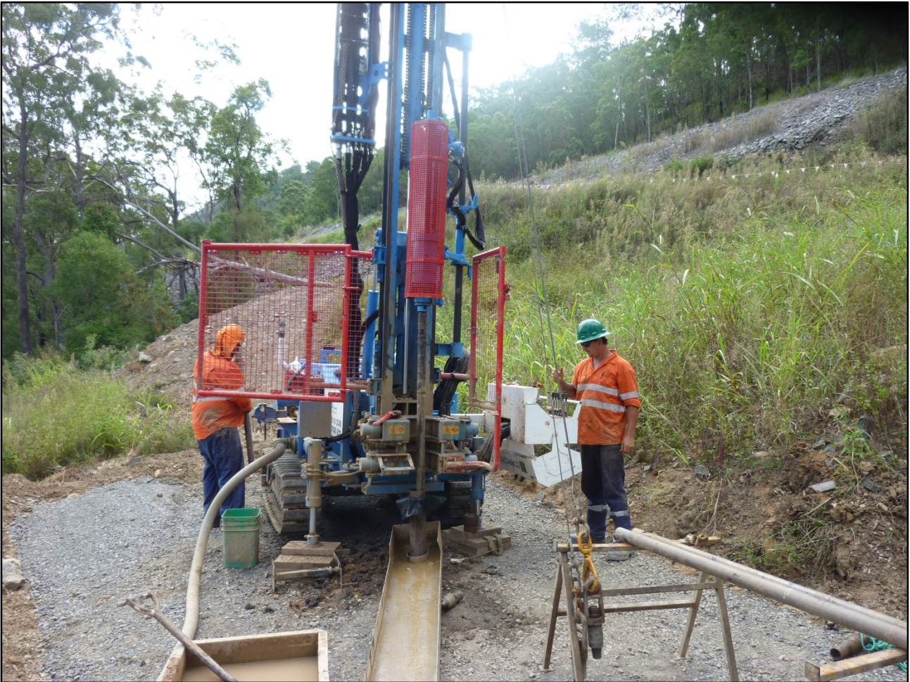
Photograph 9: View west showing drilling at Borehole BH08 within the landslip zone at approximate Ch 144.55 km.
