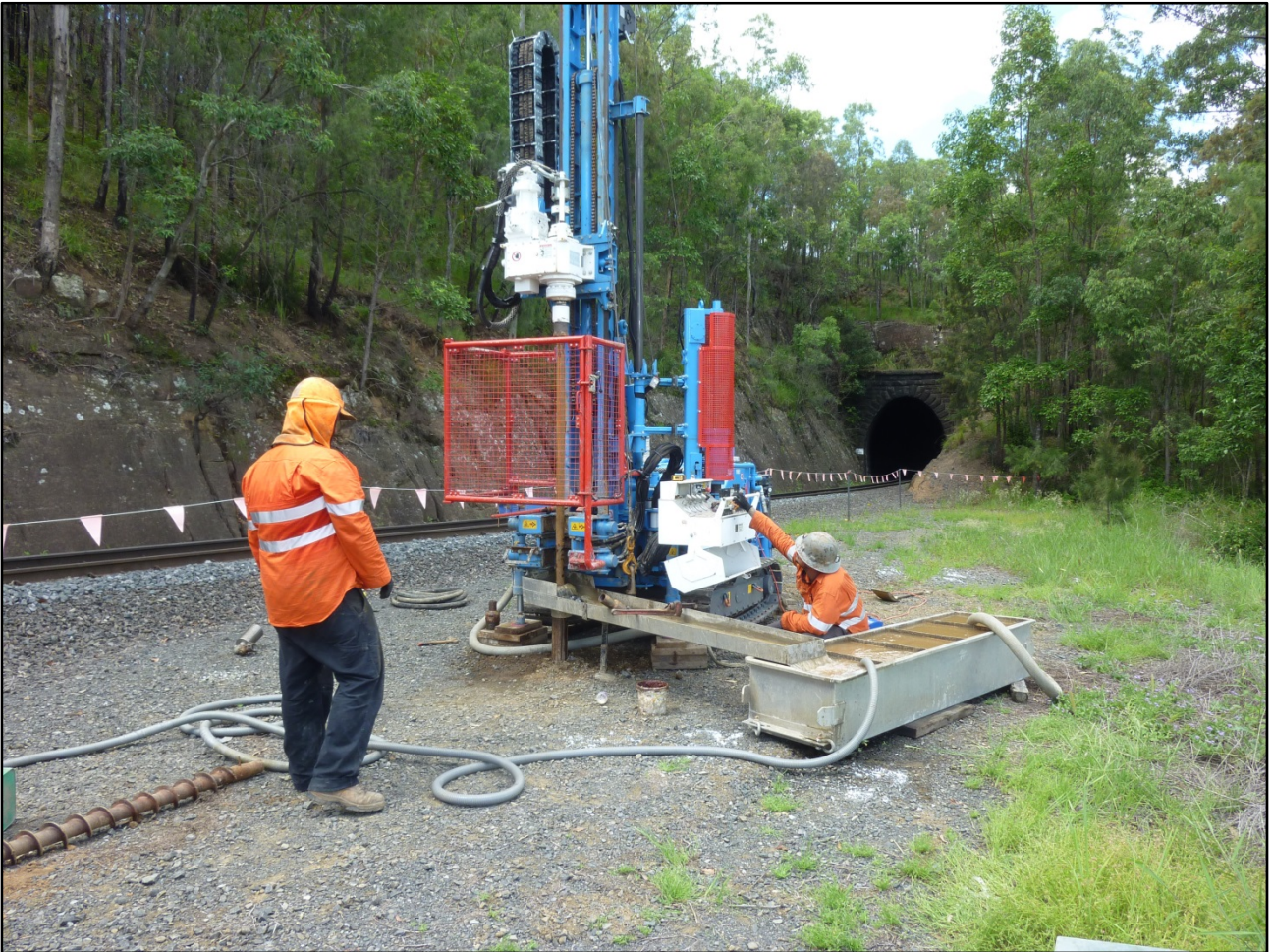
Photograph 1: View east showing drilling at Borehole BH07 on the upper access road at approximate Ch 144.57 km, with Tunnel 3 visible in the background. Note: in situ distinctly weathered sandstone exposed in the upslope cutting adjacent to the rail line.
