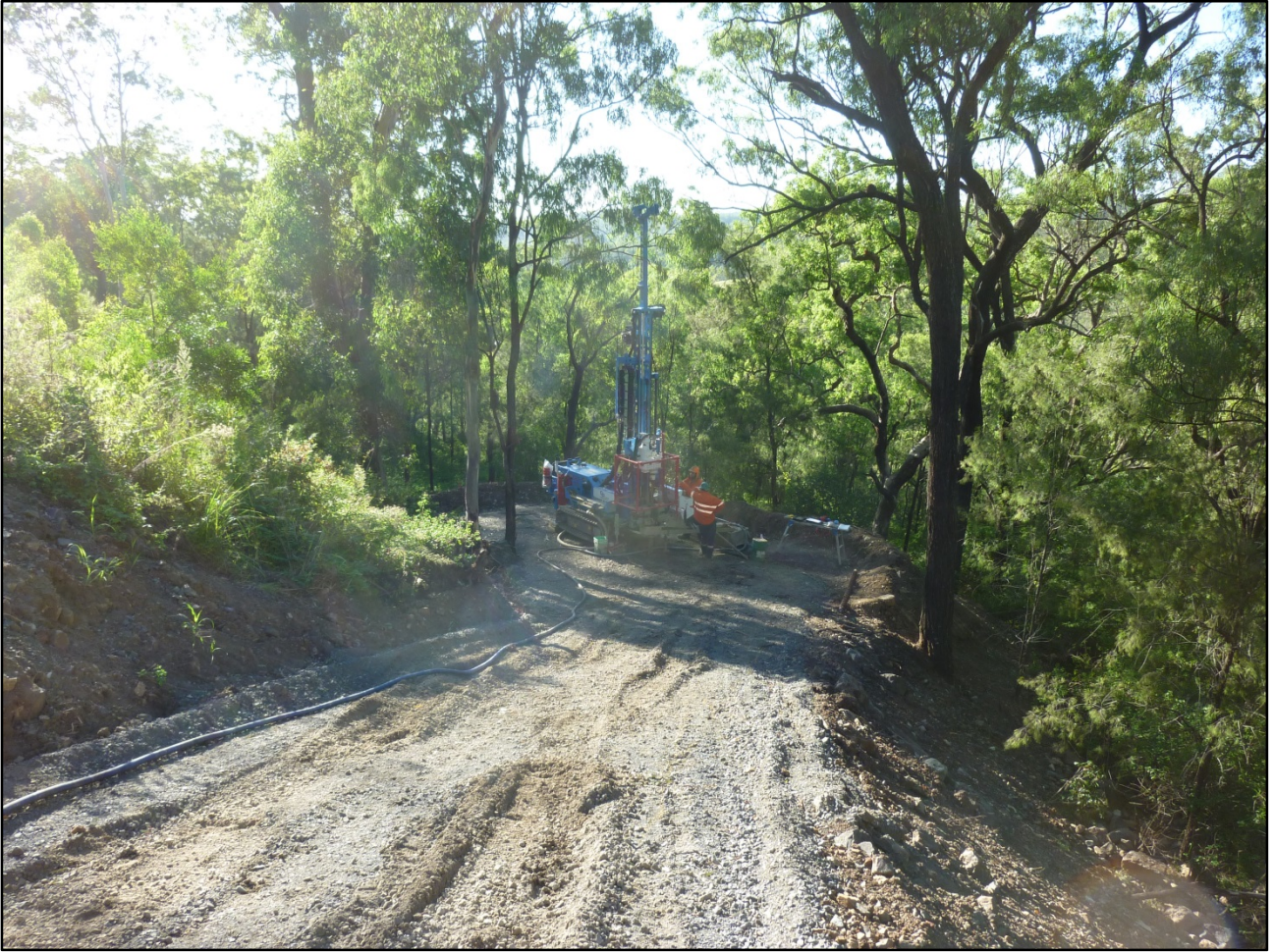
Photograph 6: View south-east showing drilling at Borehole BH04 (approximate Ch 144.7 km).
