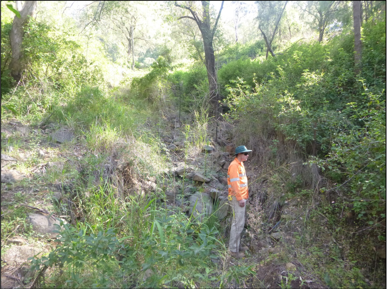
Photograph 5: View north-west at Geological Observation point G2 (located downslope of Borehole BH02) showing a gully filled with colluvium comprising predominantly basalt cobbles and boulders. This gully is the outflow channel for the under-rail culvert located at Ch 144.92 km.
