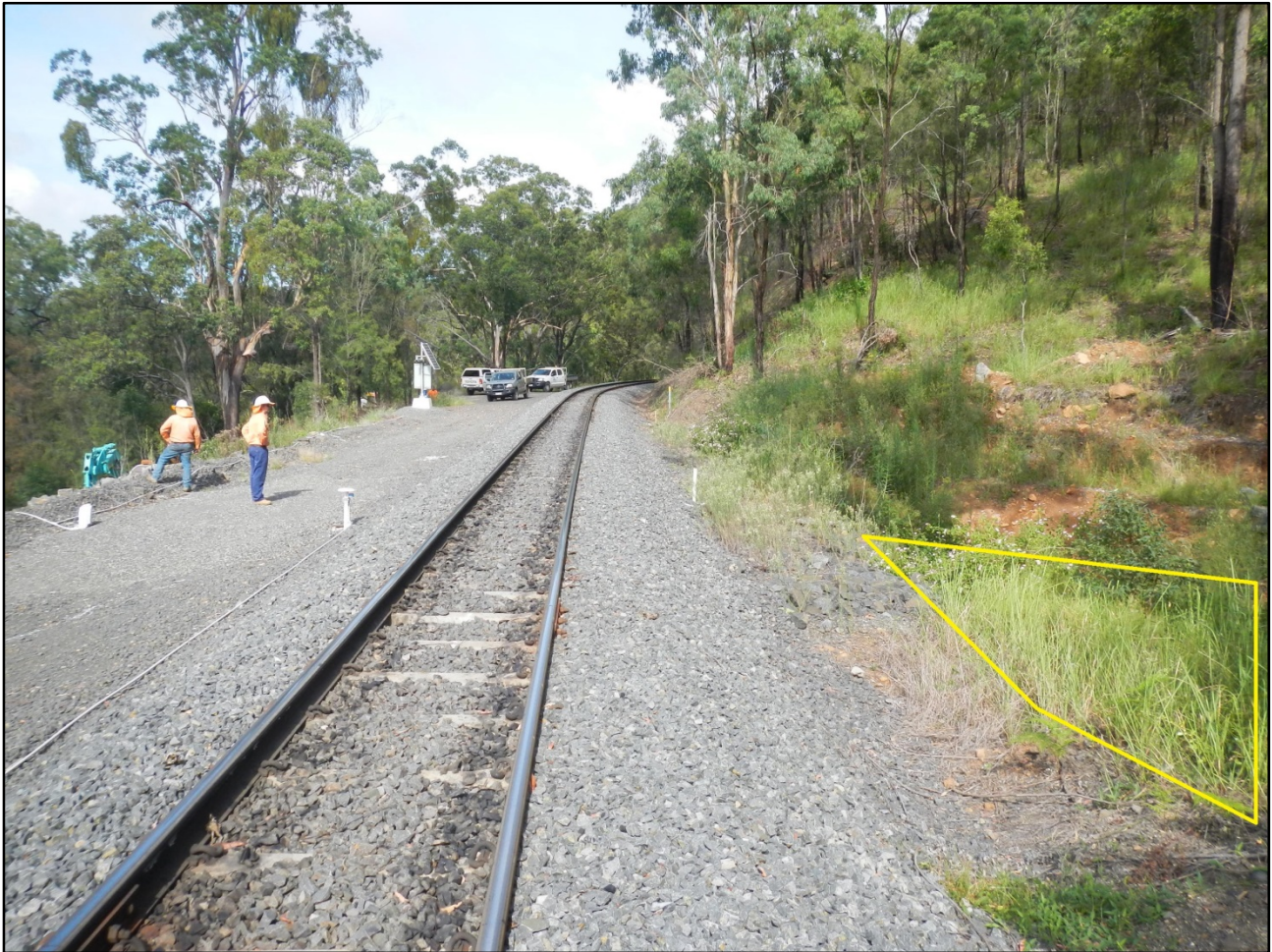
Photograph 2: View west along the railway corridor showing the upper access road and rail line at approximate Ch 144.7 km (near Borehole BH03). The inlet area for the under-rail culvert at Ch 144.73 km is visible in the right foreground of the image (marked in yellow).
