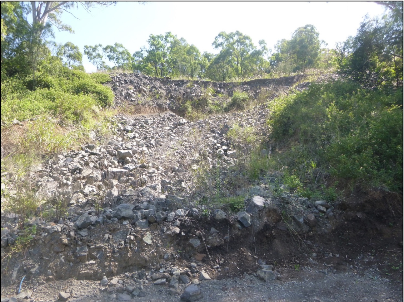
Photograph 2: View north (from location of Borehole BH02) showing landslide between approximate Ch 142.700 km and Ch 142.725 km with 7 m vertical failure scarp visible at slope crest adjacent to the access road.
