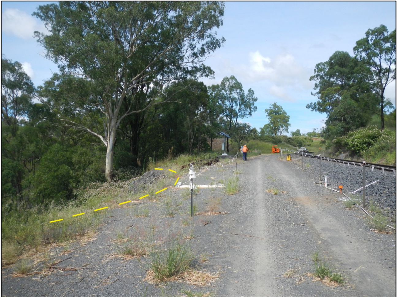
Photograph 1: View south-west along the railway corridor at Ch 142.7 km showing the landslip failure scarp (dashed yellow line), access road and rail line.
