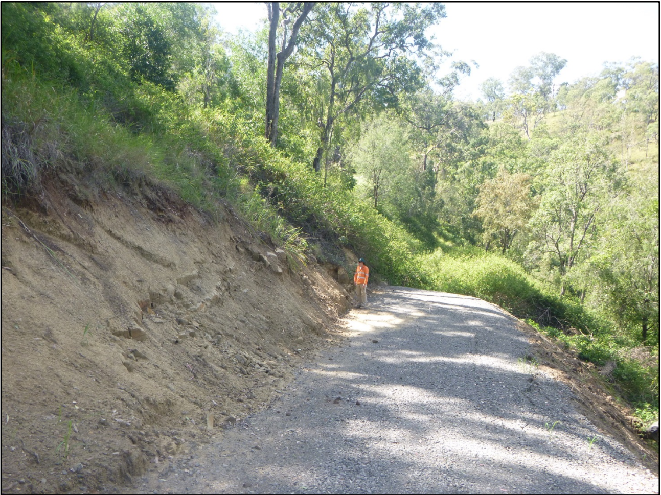
Photograph 4: View north-east showing the temporary access track at the location of Borehole BH04 and in situ extremely to distinctly weathered mudstone with interbedded sandstone layers exposed in the upslope cutting.
