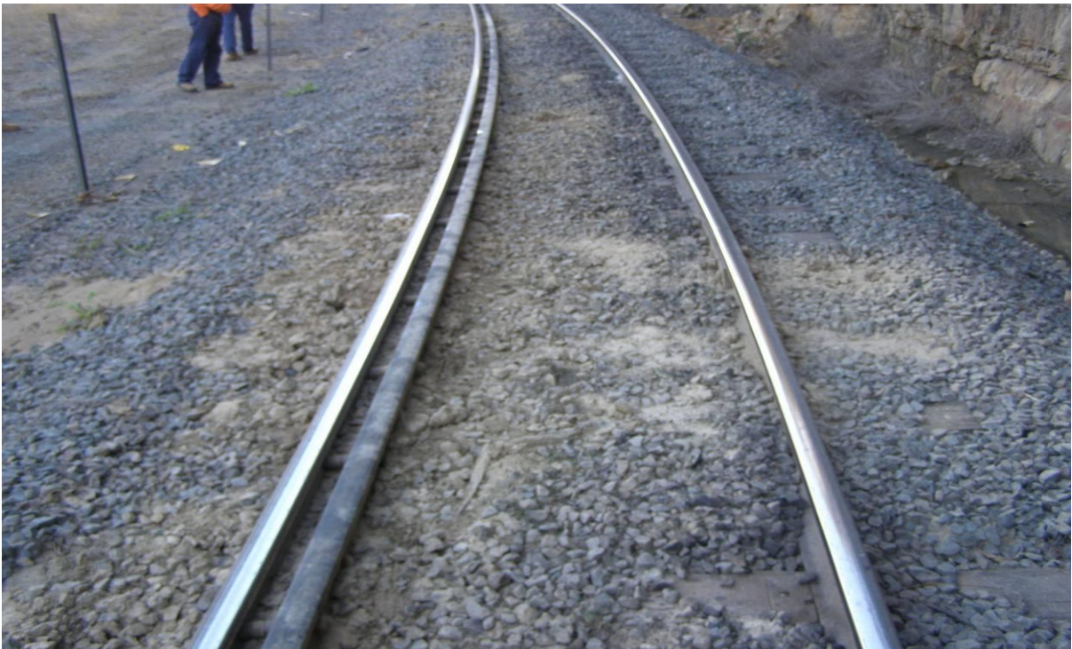
Figure 6 Existing curve with check rail (and mudhole)
