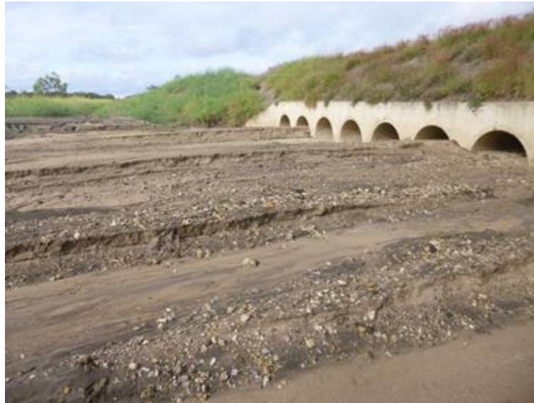
Figure 19 Pipe silting in the Newlands system
