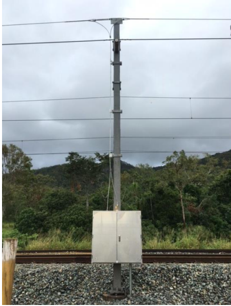
Figure 13 Photo taken following works
