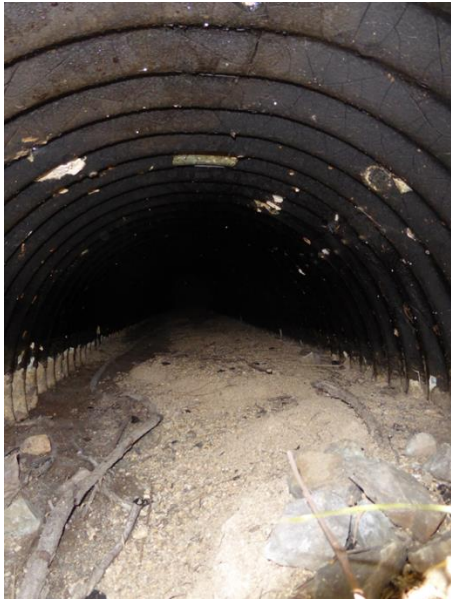
Figure 14 Goonyella Culvert CH42.96, 2016
