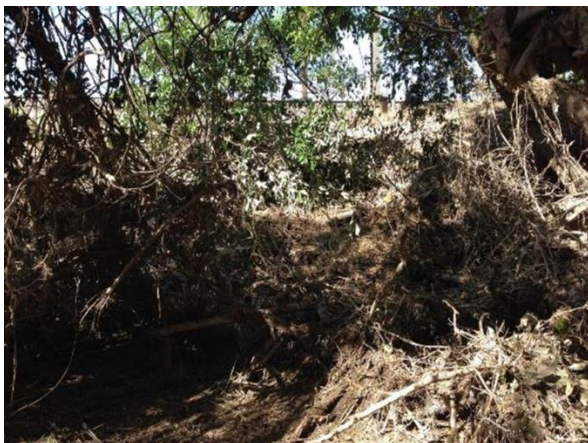
Figure 16 Goonyella Culvert CH44.70, after TC Debbie
