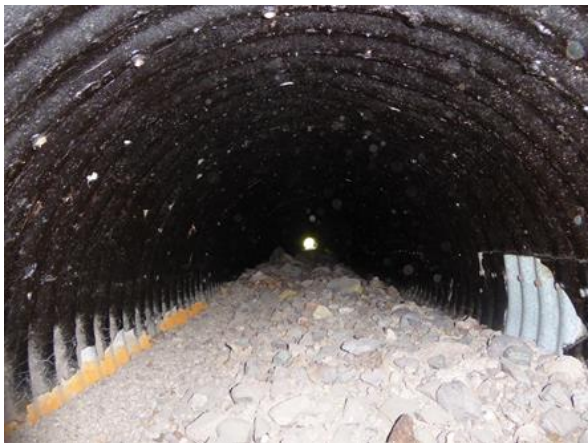
Figure 15 Goonyella Culvert CH44.70, 2016
