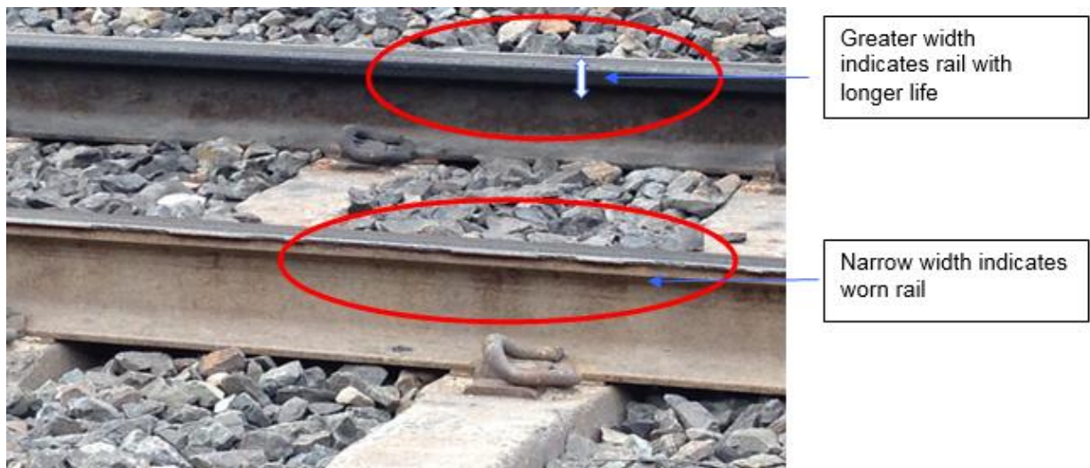
Figure 3 – Rail wear
