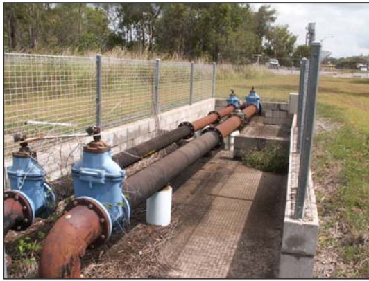
Orica Metered Service Connection with By-pass – Satisfactory Condition
