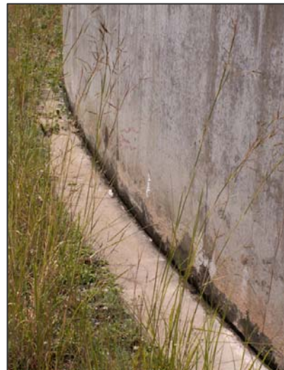
Mt Miller Reservoir – Wall / Floor Seal – good condition
