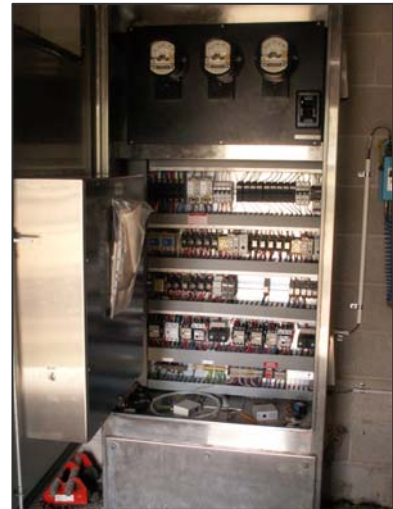
Wilmott PS Electrical Switch Board – Good condition
