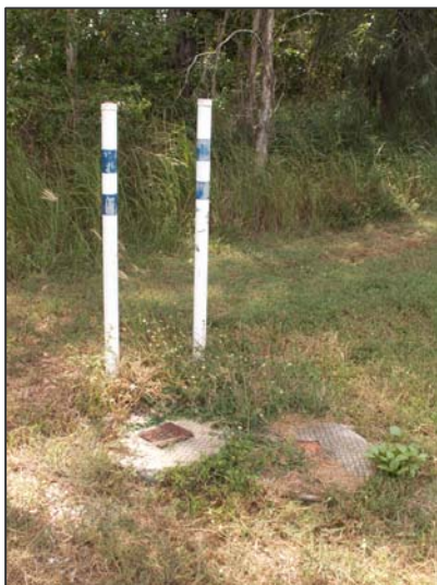
Typical 20mm Temporary Service Connection – Good condition
