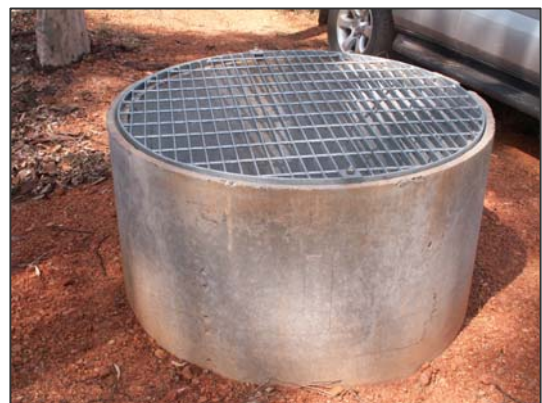
Typical New Air Valve Pit – As new
