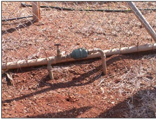
Typical 20mm Temporary Service Connection – Good condition
