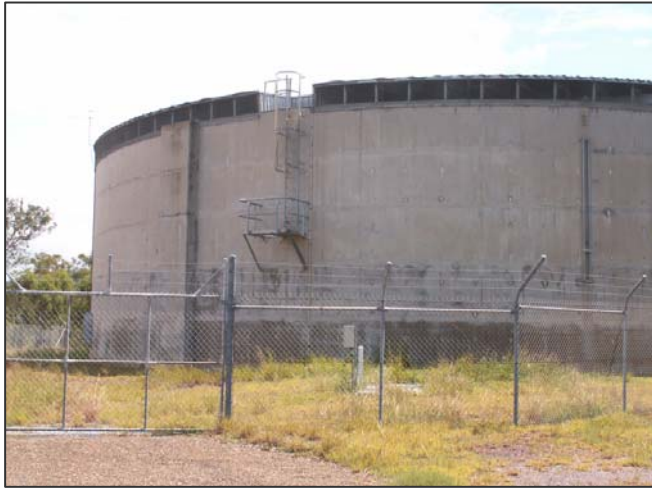
Mt Miller Reservoir (including security fencing & access ladder) – good condition
