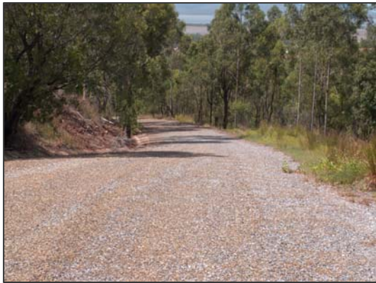
Mt Miller Reservoir – Access Road Well maintained & good condition
