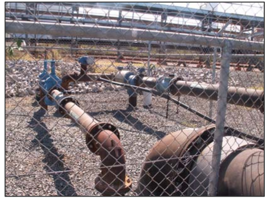
Comalco Service Connection, By-pass & Raw Water Supply – Good Condition
