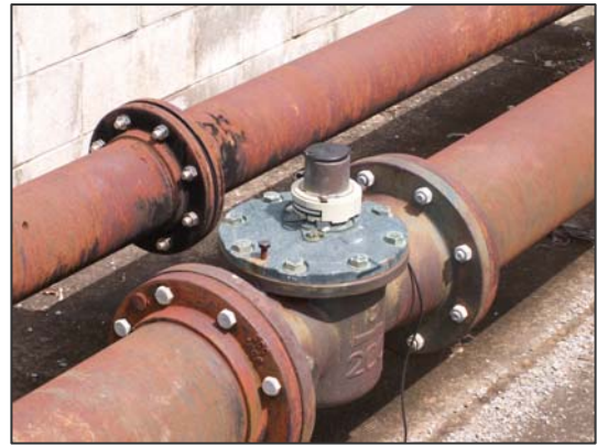
Orica 200mm Meter – Satisfactory Condition
