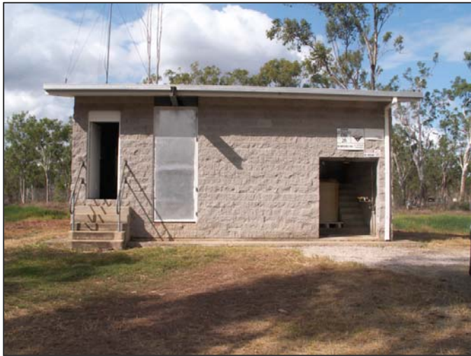
Wilmott Pumping Station (PS) & Chlorinator – Good condition
