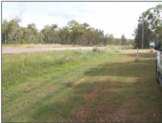
Typical Road Pipeline Location & Access – Well maintained
