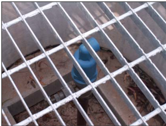
Typical New 50mm Air Valve – As new
