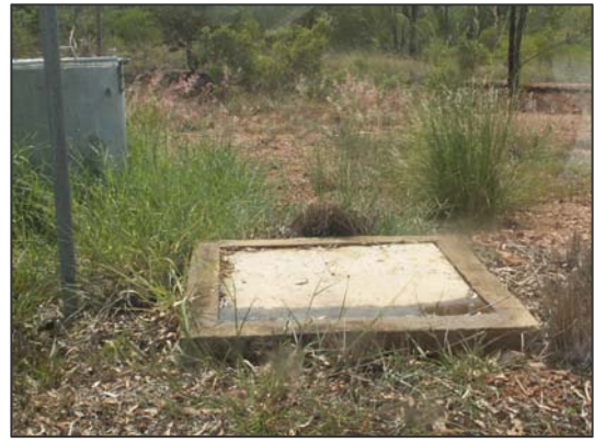
Typical Older Style Scour and Valve Pit – Good condition
