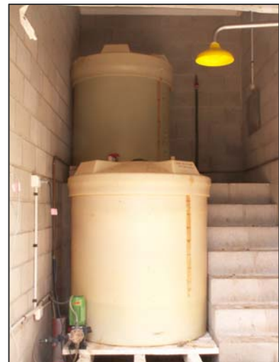
Wilmott Chlorinator Storage Tanks, Dosing Pump & Safety Shower - Satisfactory condition
