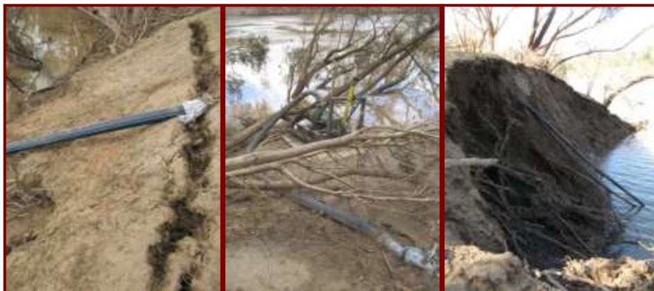
Photographs: Damage caused by Seqwater floodwater releases, Pine Mountain
