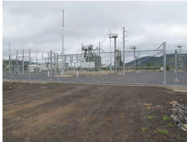
Figure D-A 1 Photo 201 – Ch 173.207
