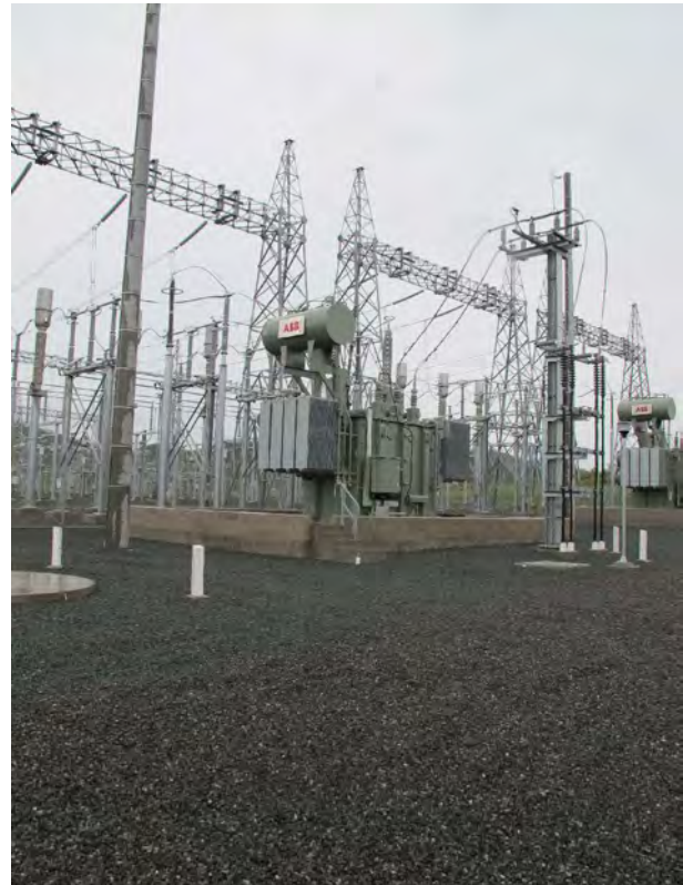
Figure D-A 73 Photo 184 – Ch 582.481
