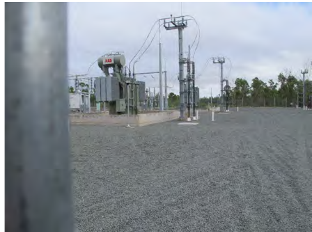
Figure D-A 9 Photo 200 – Ch 103.847
