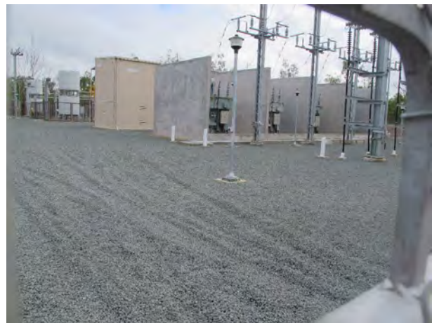
Figure D-A 8 Photo 199 – Ch 103.847
