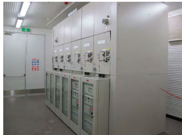
Figure D-A 13 Photo 197 – Ch 49.200
