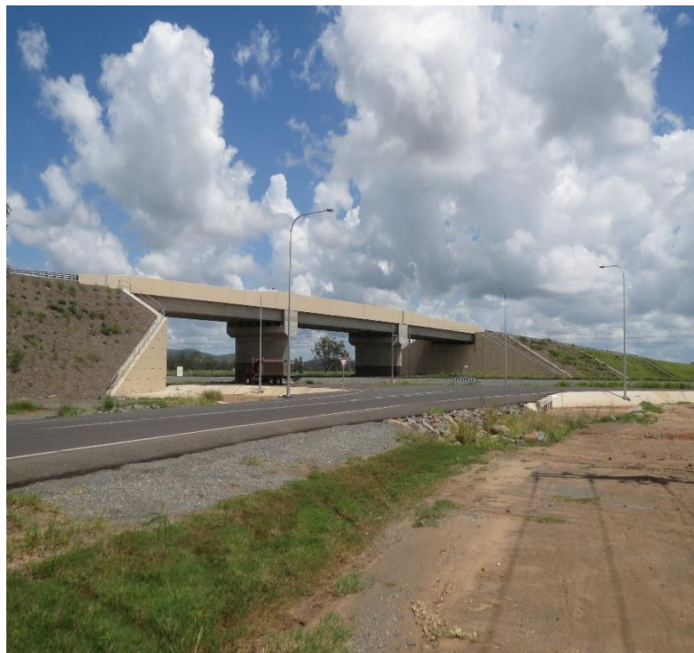
Figure 4-1: Gracemere overbridge – TACA
