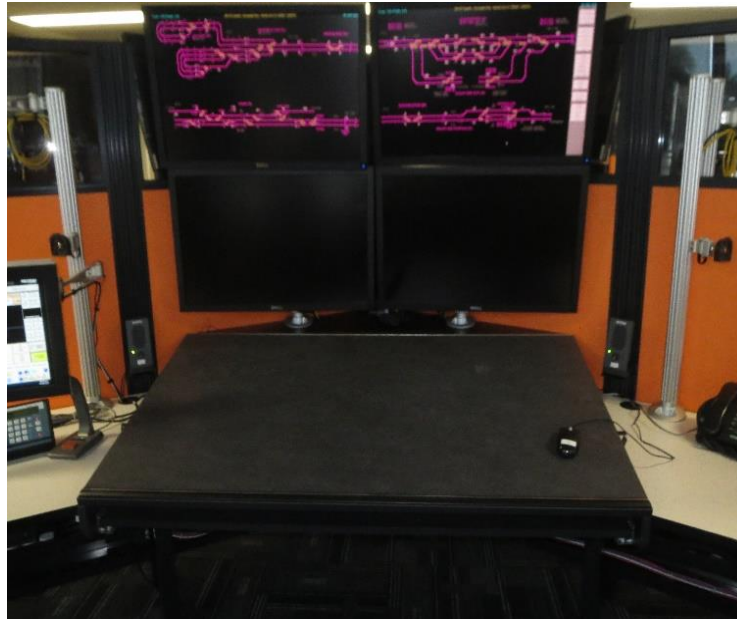
Figure 5-3: Controller work station, Mackay Facility
