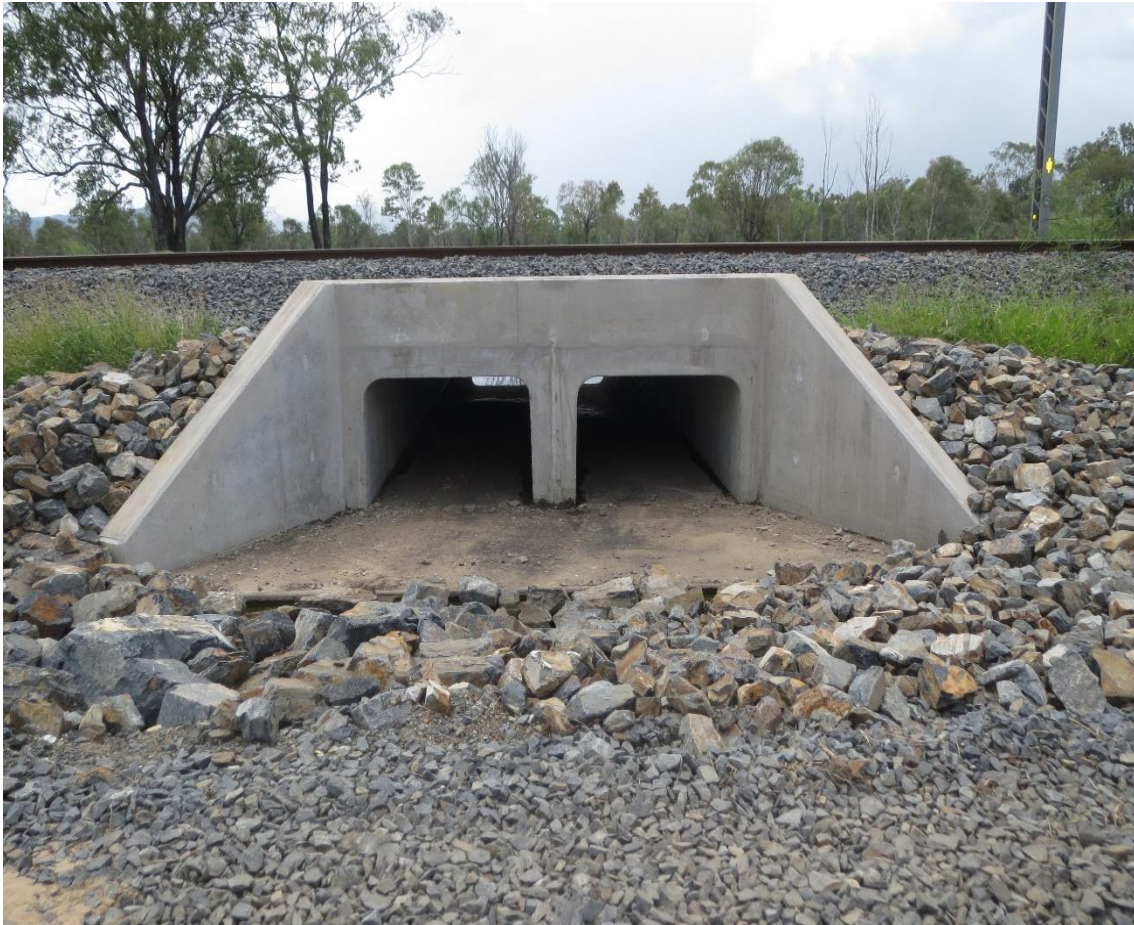
Figure 4-2: Typical culvert renewal works
