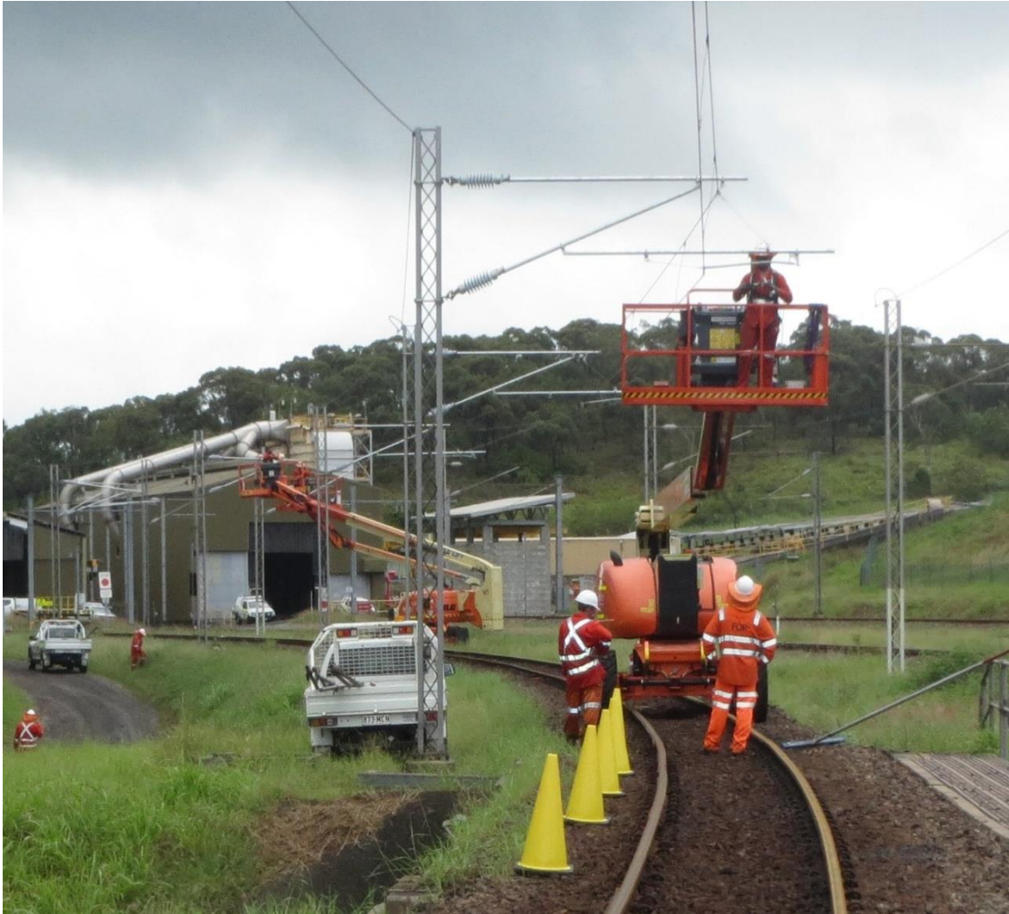
Figure 4-3: Overhead equipment works
