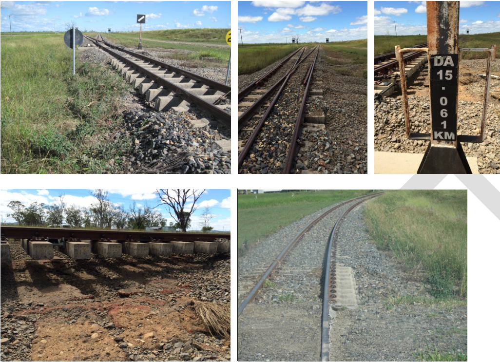
MSL69 – During re-instatement works
