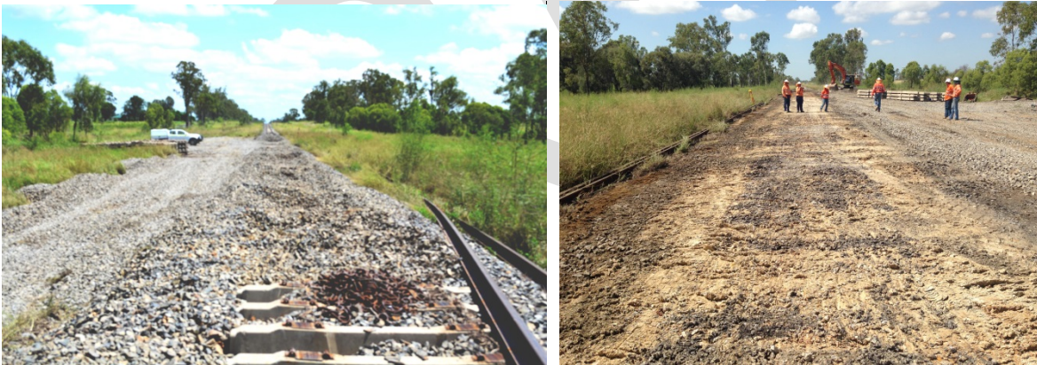
MSL66 – During re-instatement works. Removal and reinstatement of 200 m of rail, ballast and formation.
