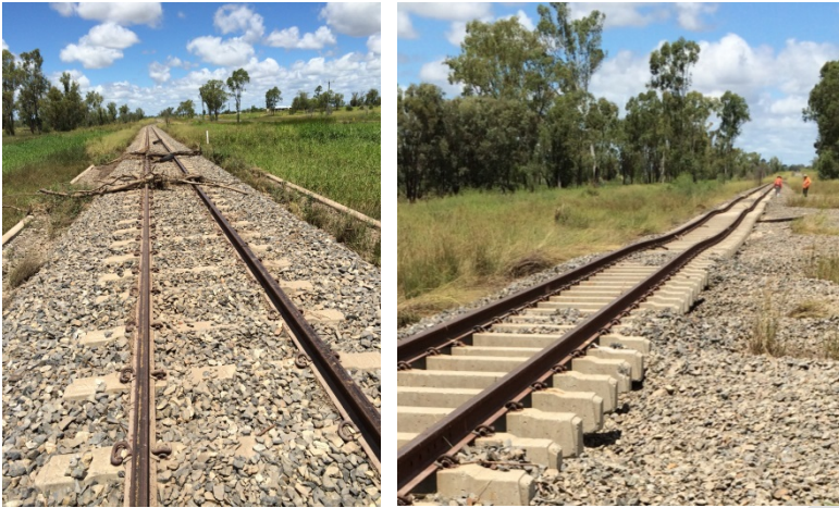
MSL66 – After the Flood, before re-instatement works
