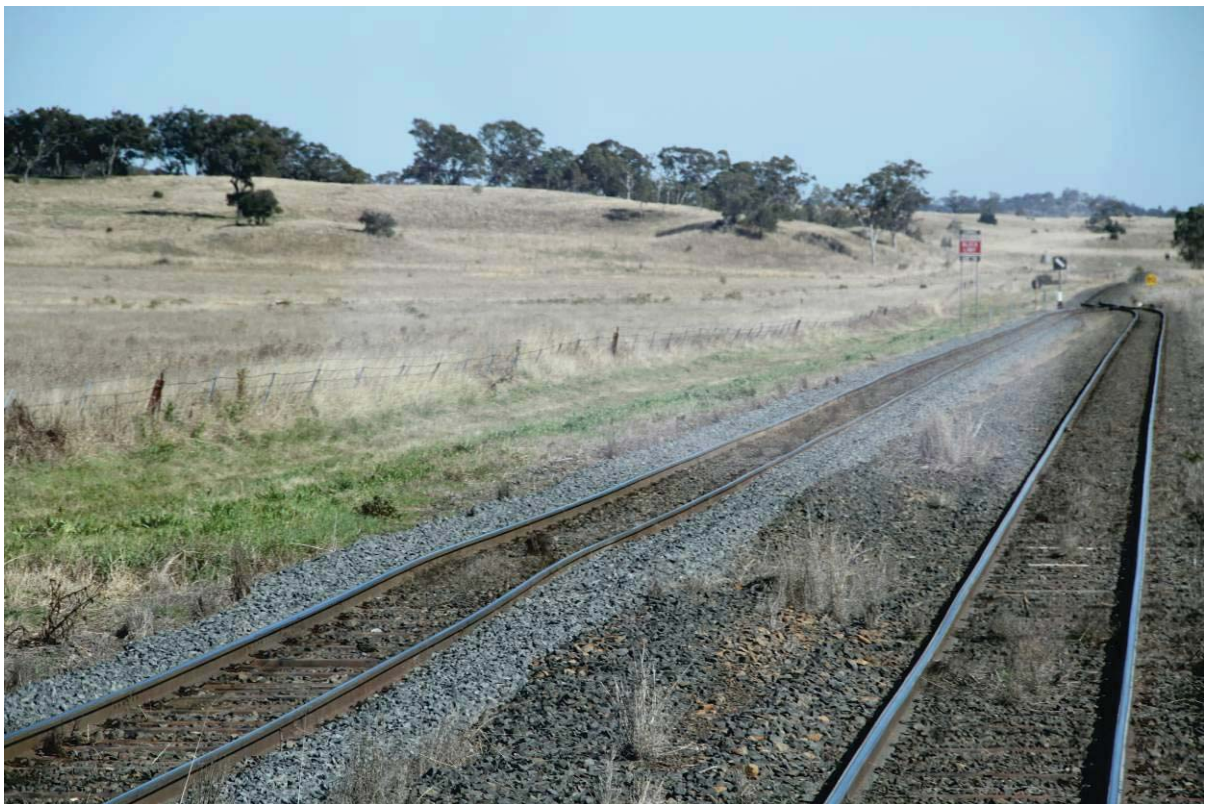
Figure 35 - Dip in top and line due to loss of structure integrity
