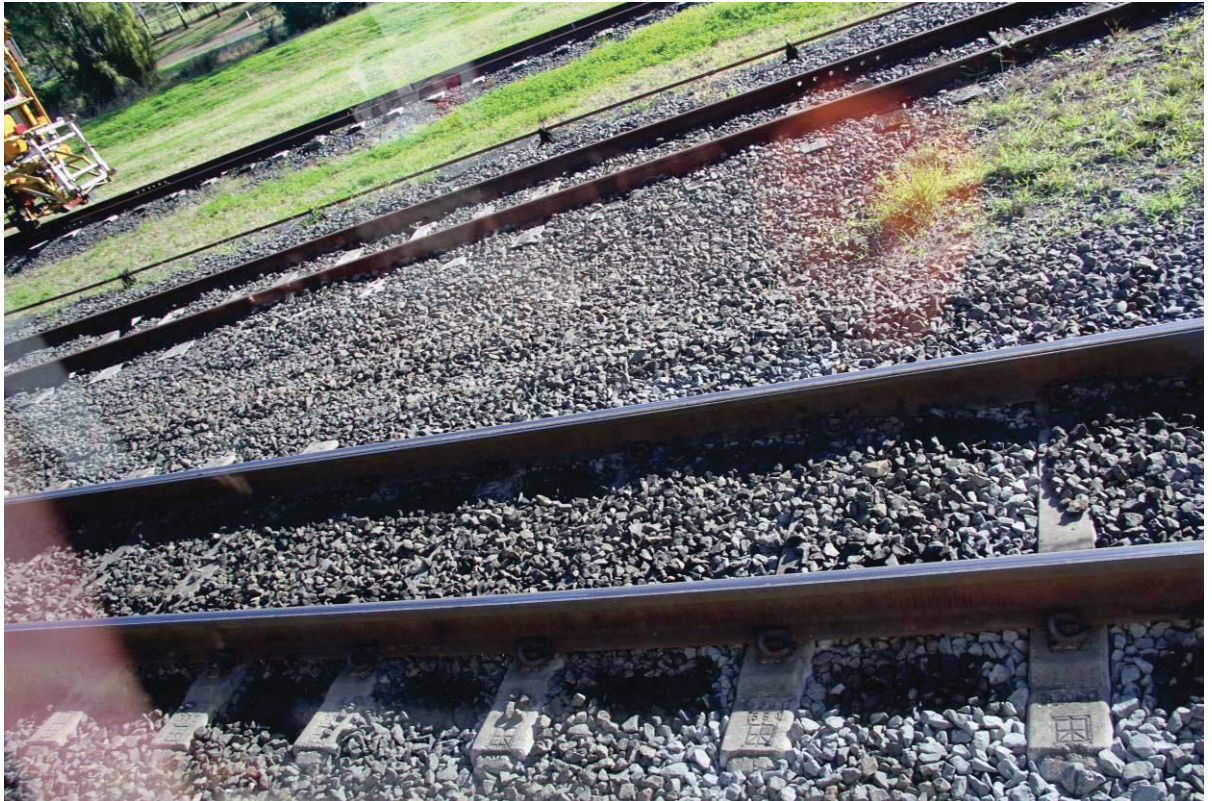
Figure 22 - Typical 50 kg rail on concrete sleepers
