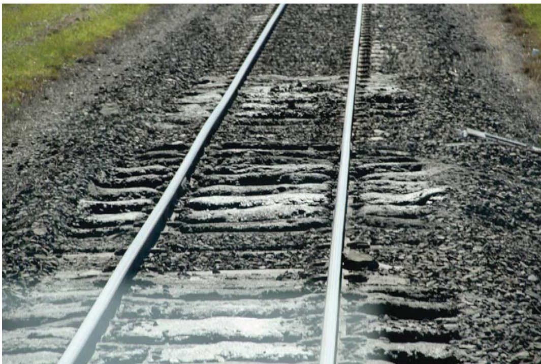
Figure 39 - Typical mudholed section
