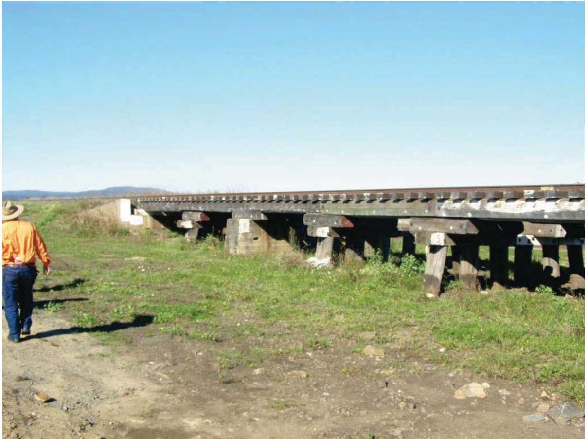
Figure 10 - Typical timber bridge (83.190 km ML)
