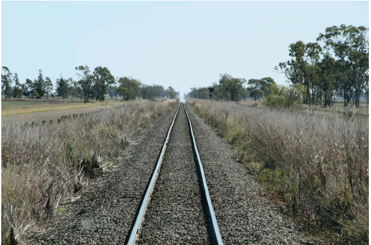
Figure 13 - Typical Top & Line problems west of Toowoomba
