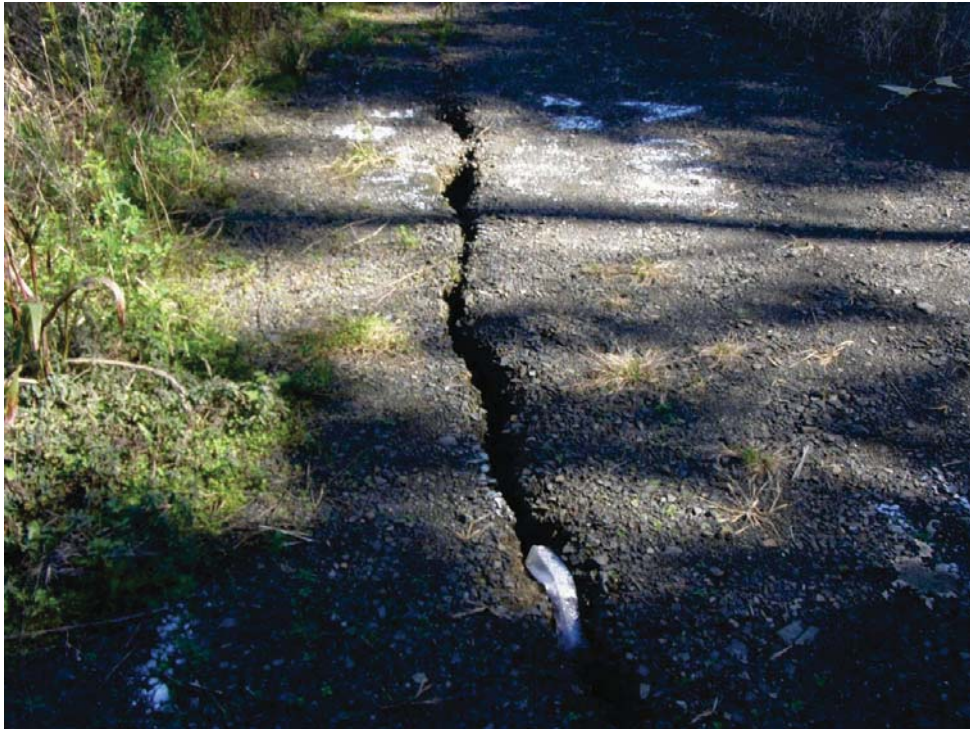
Figure 3 - Cracking on edge of access road at 144.6 km ML
