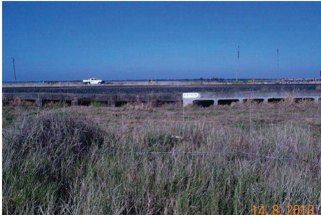
Figure 7 - Culvert at 55.270 km WL
