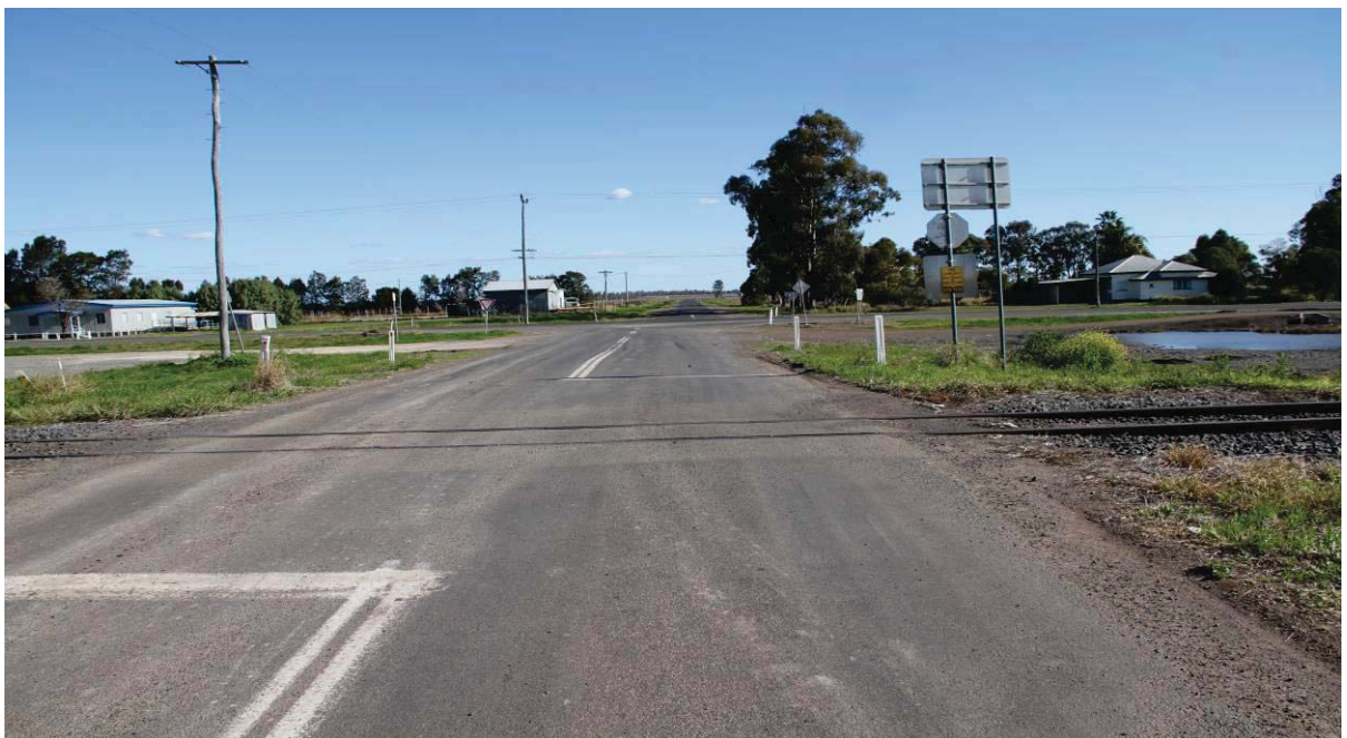
Figure 15 - Open level crossing Macalister 107.700 km WL
