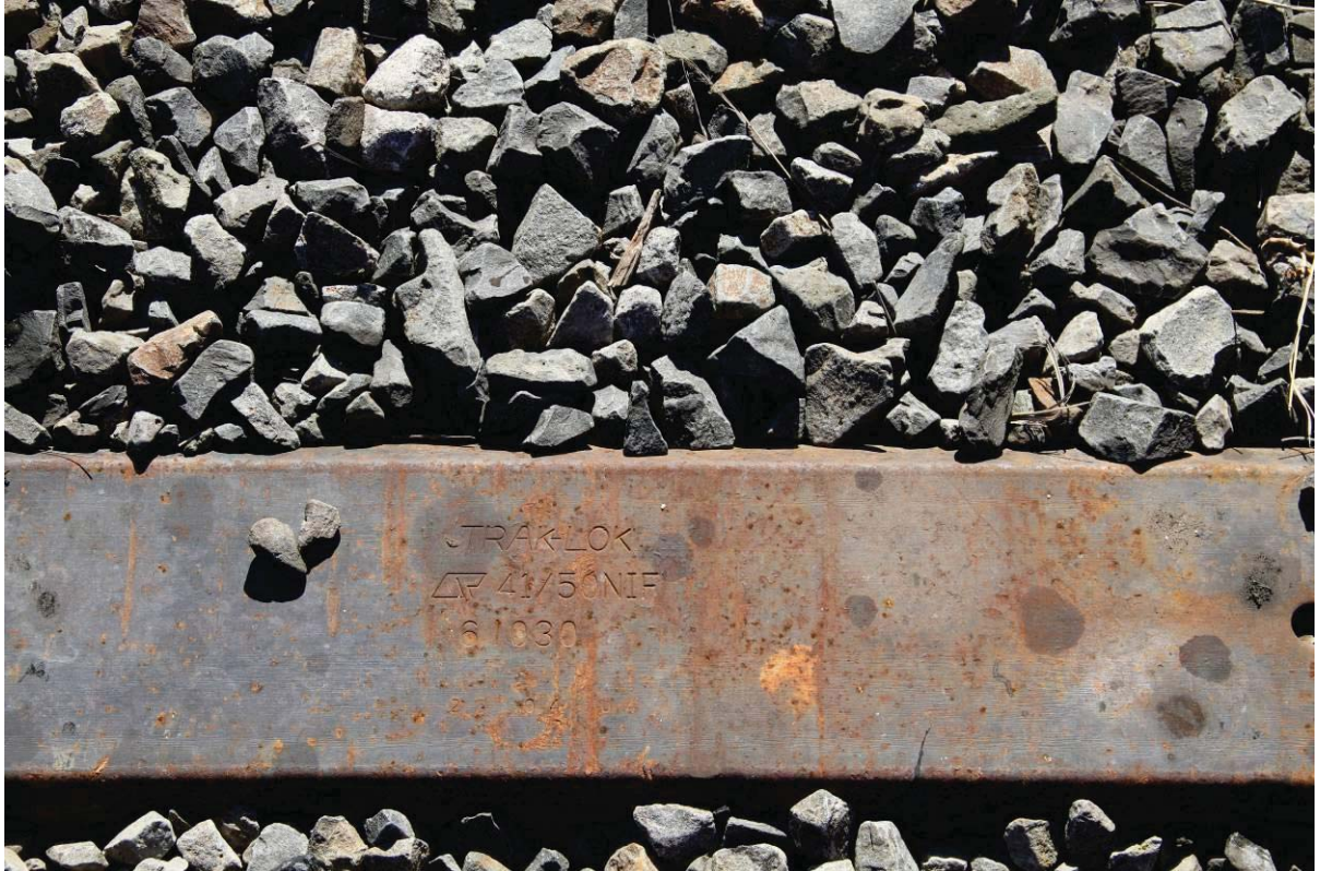
Figure 37 - Steel sleepers were generally in fair condition although some signs of corrosion and aging generally evident
