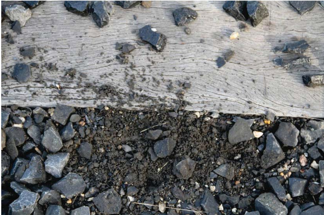
Figure 38 - Removal of top thin layer of ballast often revealed level of contamination underneath
