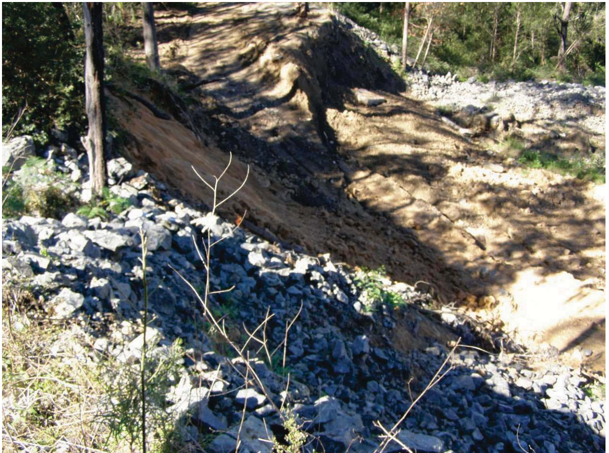
Figure 2 - Slip of face of access road embankment at 142.5 km ML
