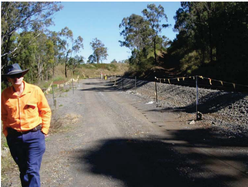
Figure 4 - Slump in access road from white post to foreground 142.5 km ML
