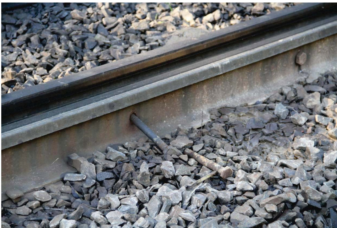
Figure 28 - Bolts protruding/snapping at checkrails
