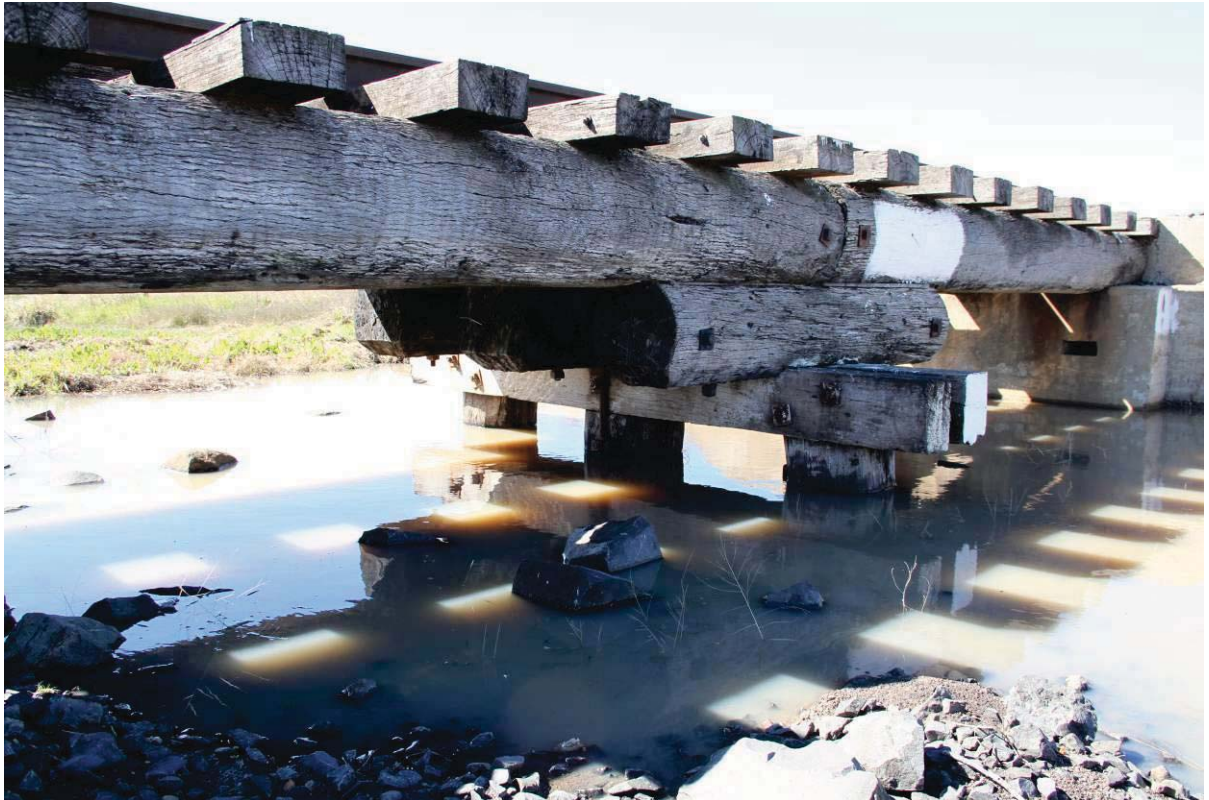
Figure 42 - Typical Timber Structure
