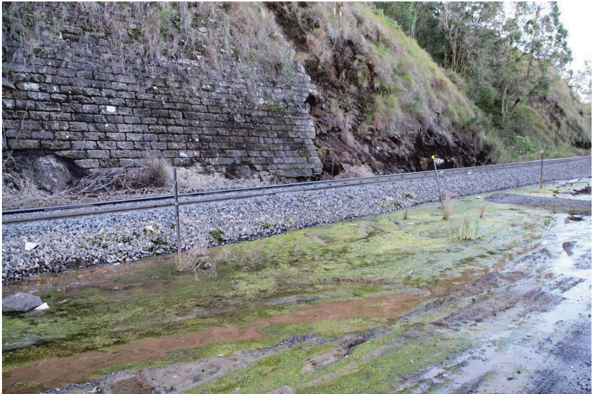
Figure 32 - An example of pooling adjacent to track
