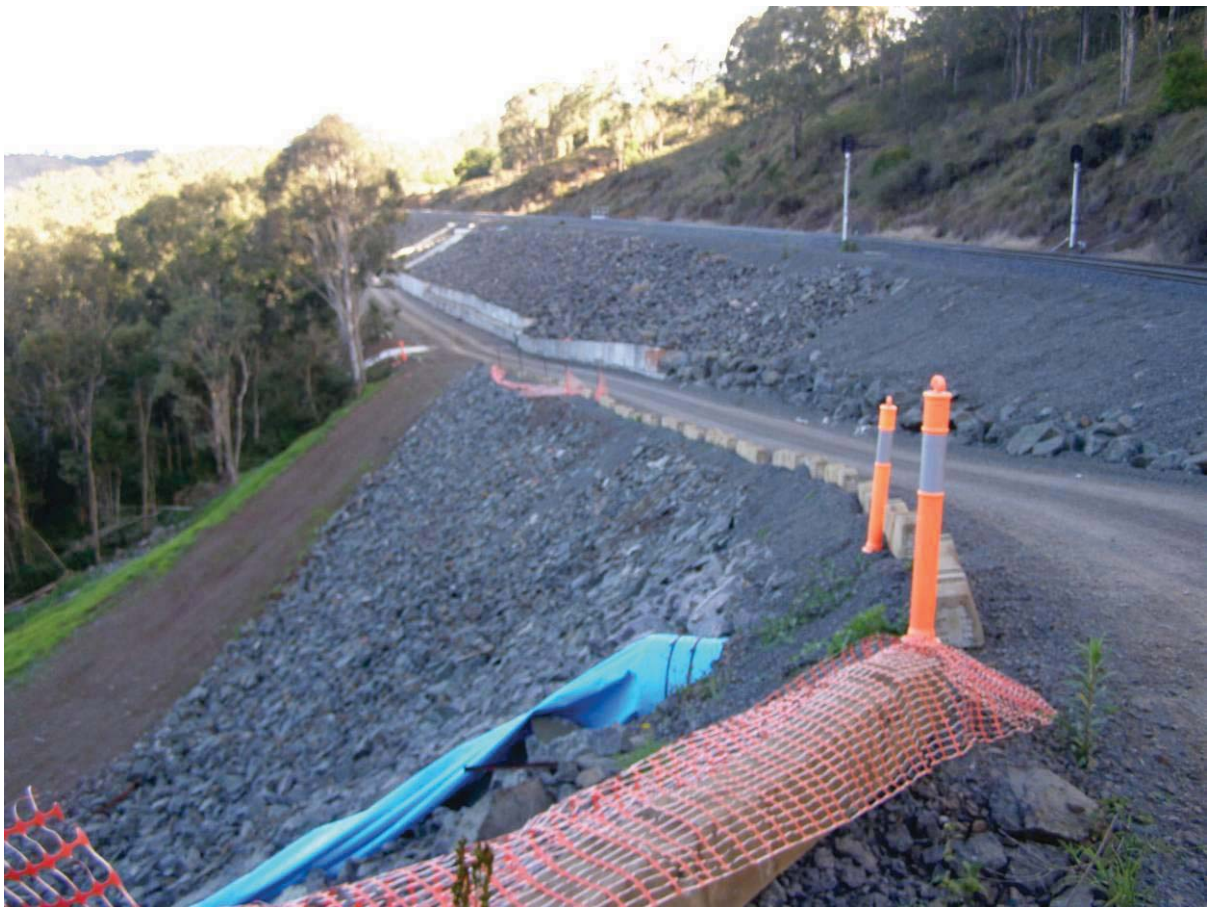
Figure 5 - Washout rectification at Rangeview 155 km ML
