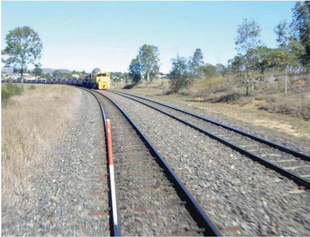
Figure 11 - Typ. 41 rail, steel & timber sleepers, plated joint, pumping
