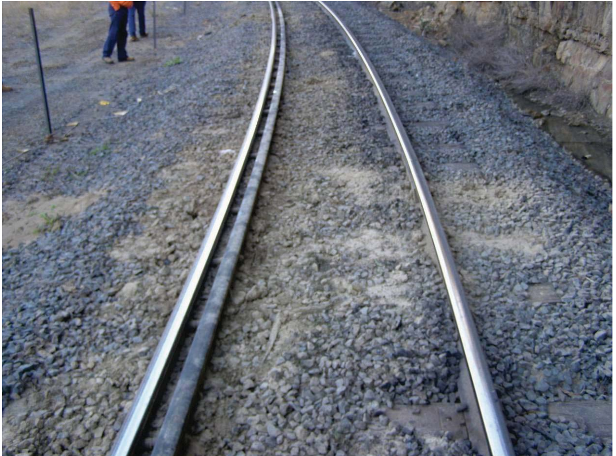
Figure 9 - Existing curve with check rail (and mudhole)
