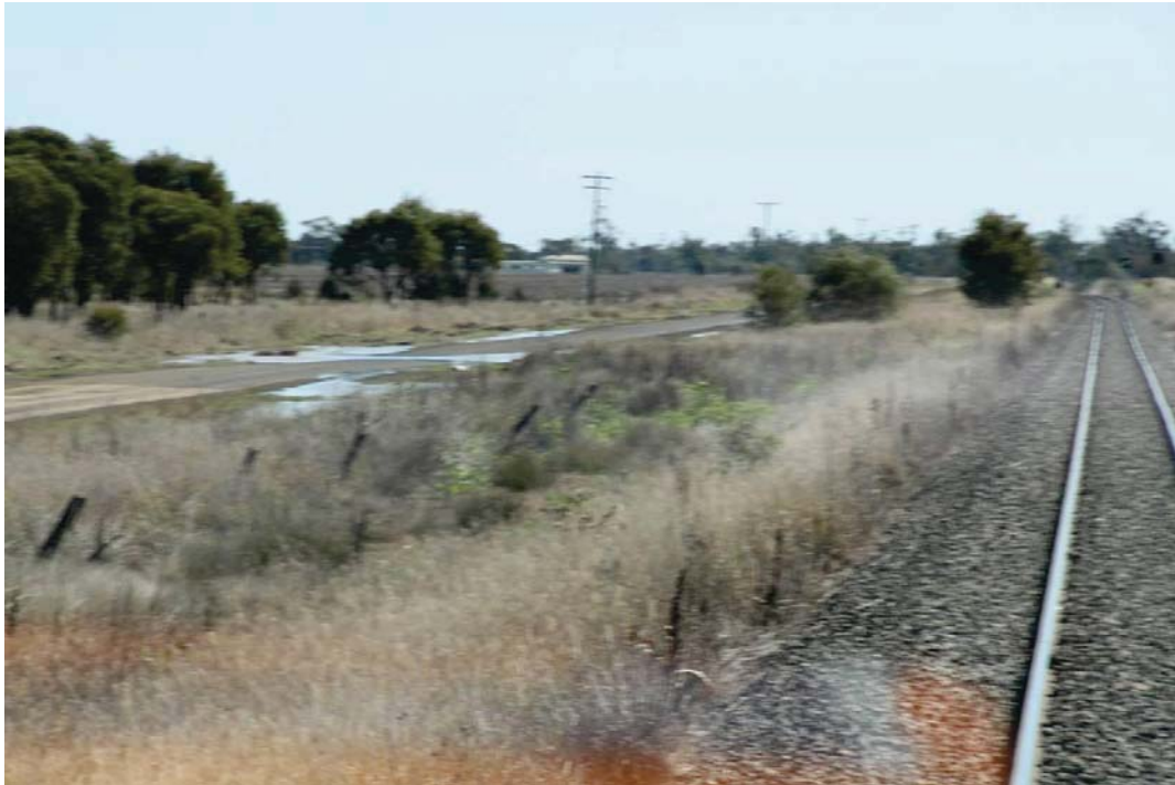
Figure 33 - Much of the adjacent highway was still flooded despite rains having stopped over 24 hours previously
