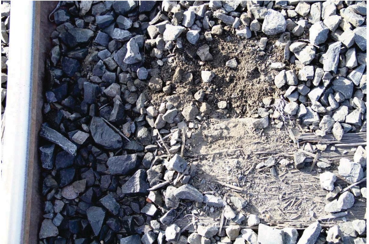
Figure 23 - Deterioration of Timber Sleepers and ballast contamination
