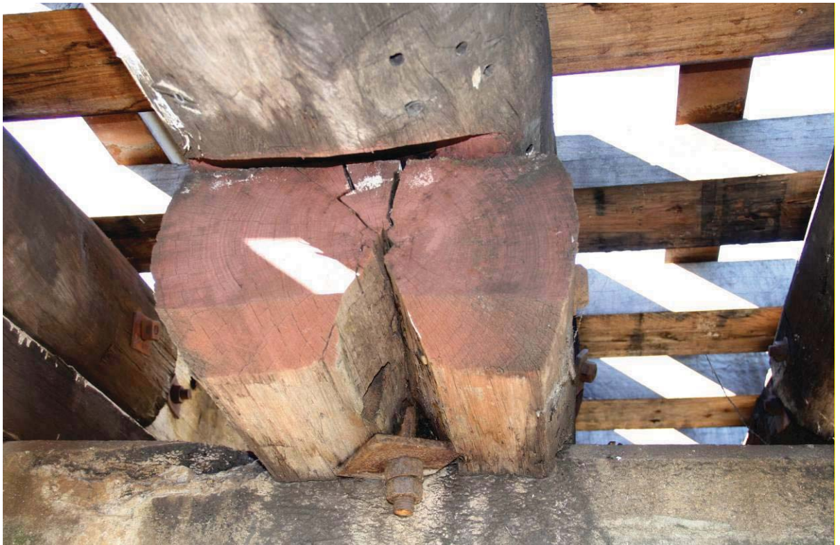
Figure 19 - Defective timbers marked for reparation
