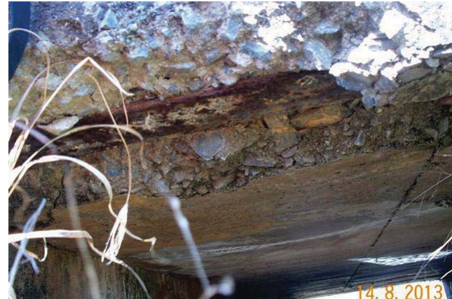
Figure 8 - Culvert at 55.270 km WL
