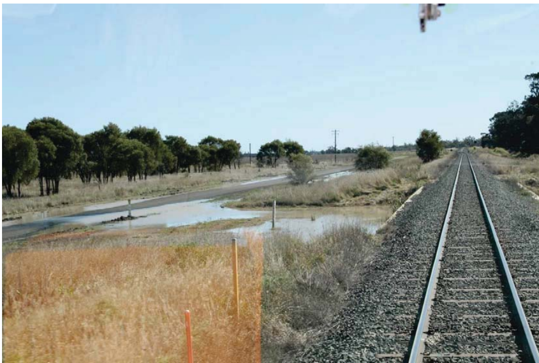
Figure 34 - Flooding and pooling of highway adjacent to culvert opening
