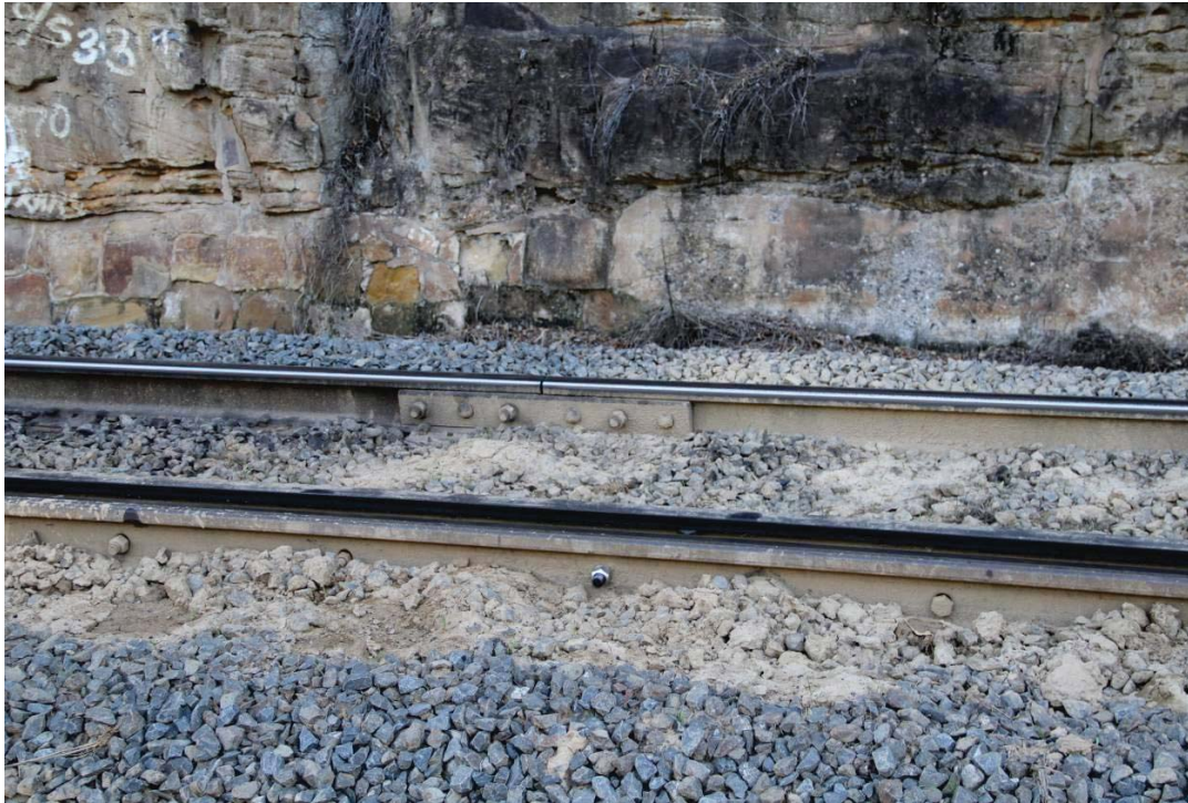
Figure 27 - Typical mudhole and evidence of bolts snapping at checkrail
