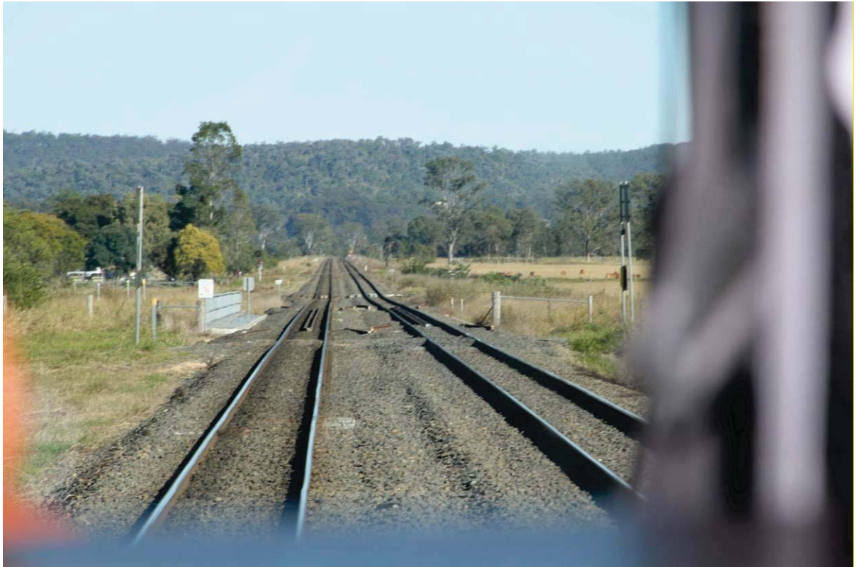
Figure 6 - Dip in Rail Track
