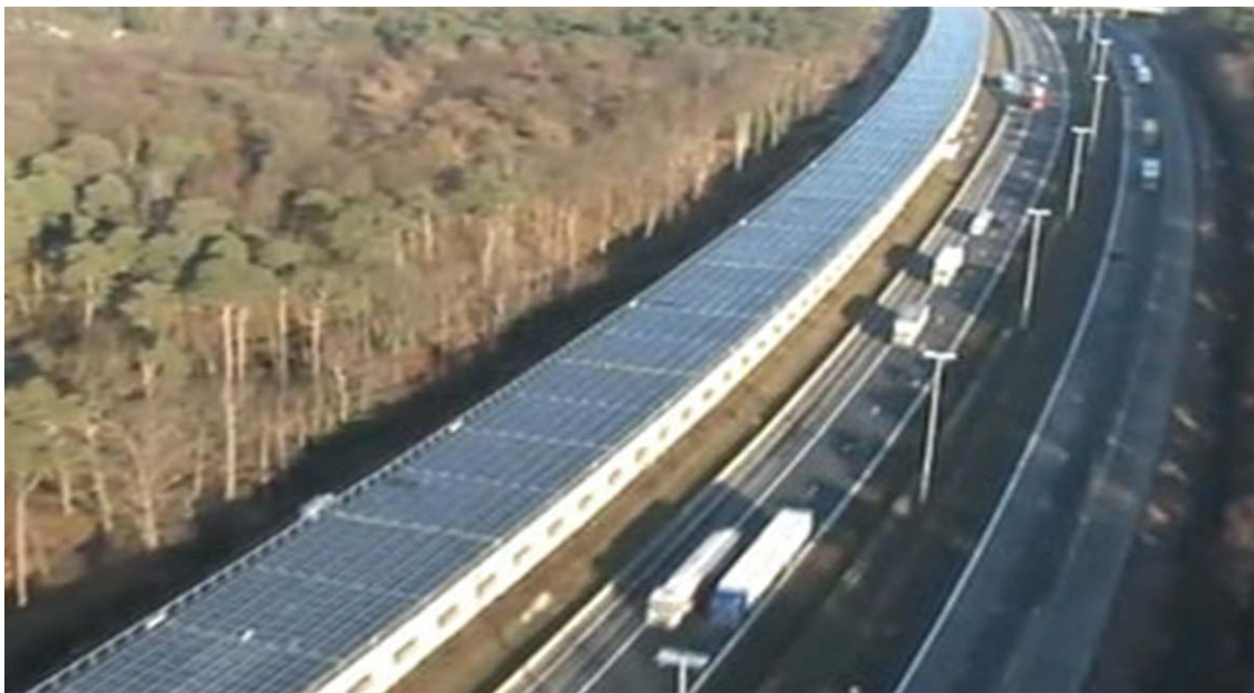
Figure 8 - The Belgian solar rail tunnel 102
