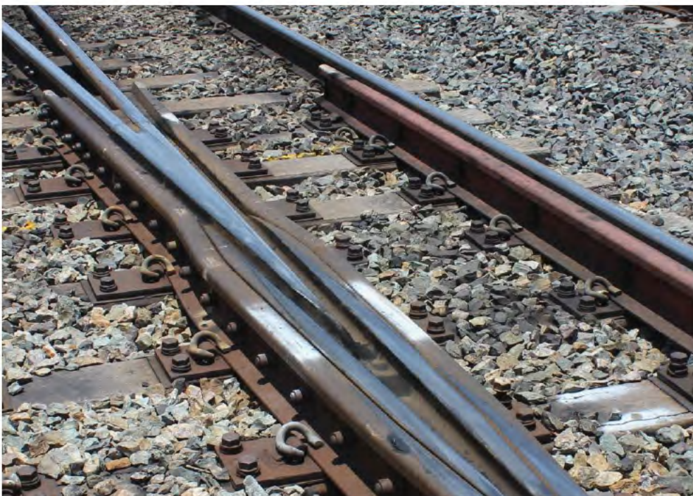
Figure 7.12: The same RBM Vee site refurbished under the FY 19 capital works
