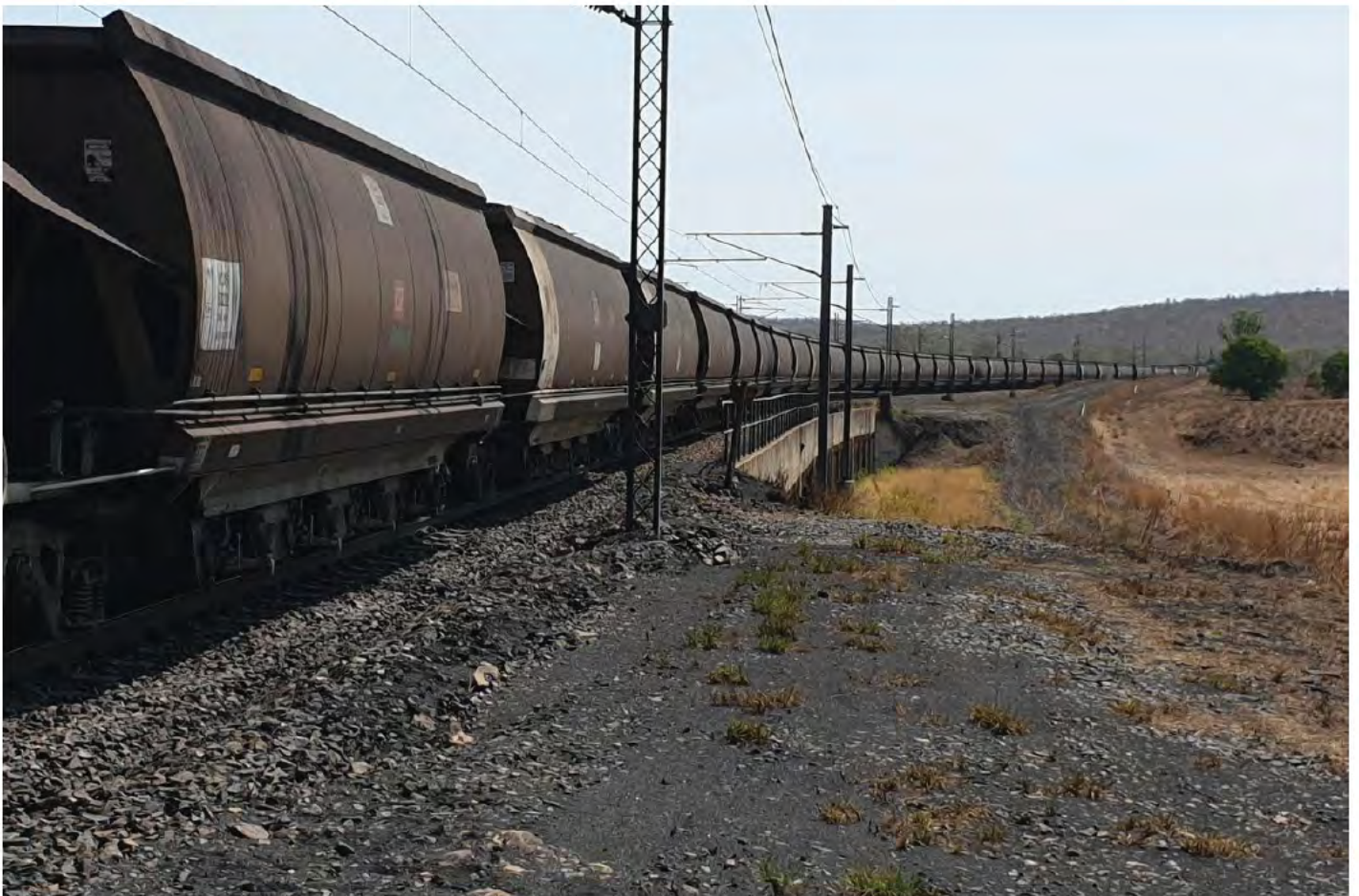
Figure 7.14: Coal dust contamination on the approach to a bridge on the Goonyella System
