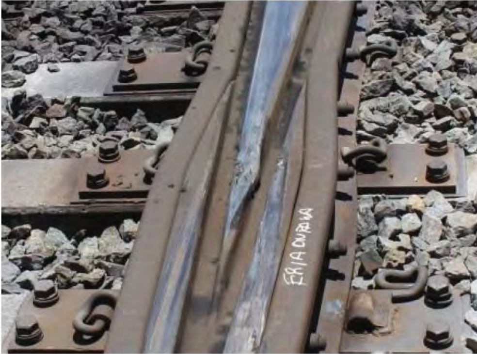
Figure 7.11: Damaged RBM Vee at Waitara in 2016 during the Condition Based Assessment
