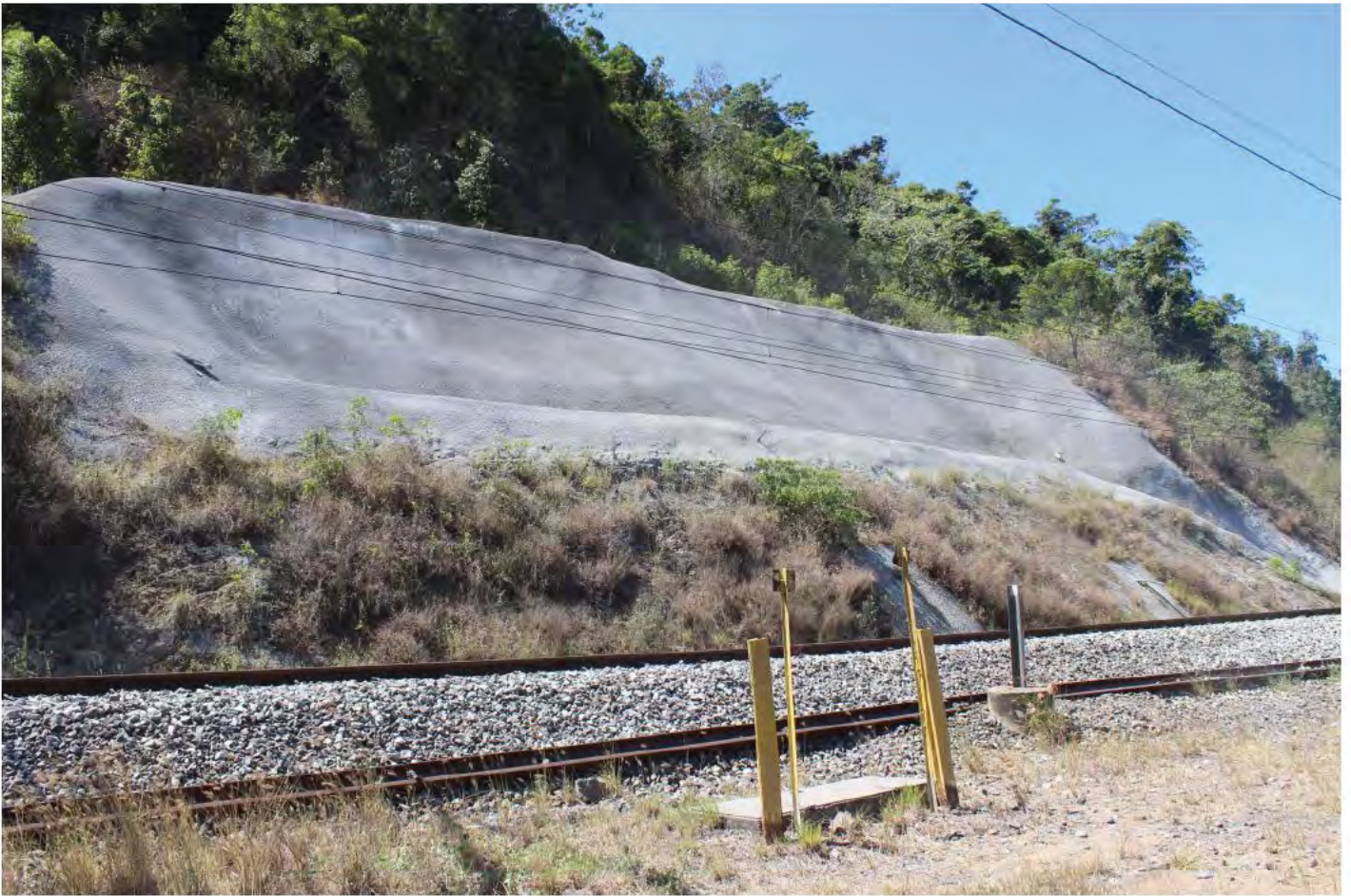
Figure 7.1 Cyclone Debbie emergency repairs - fibre reinforced shotcrete slope stability works at Black Mountain (GA 43.097)
