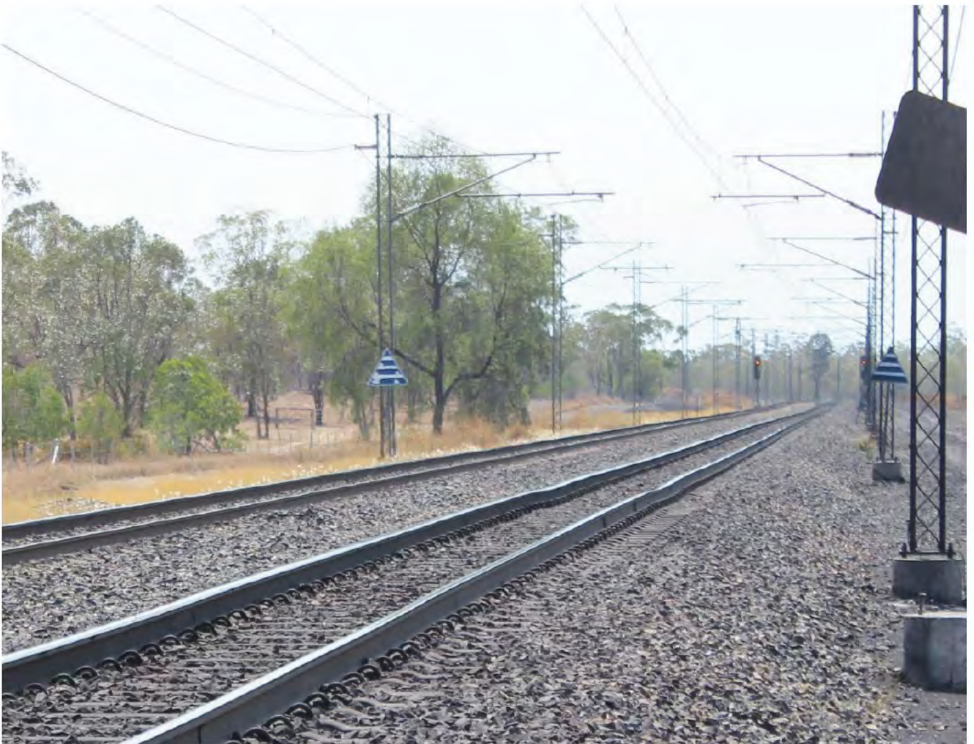
Figure 7.9: Track geometry defect west of Mindi on the Goonyella System.
