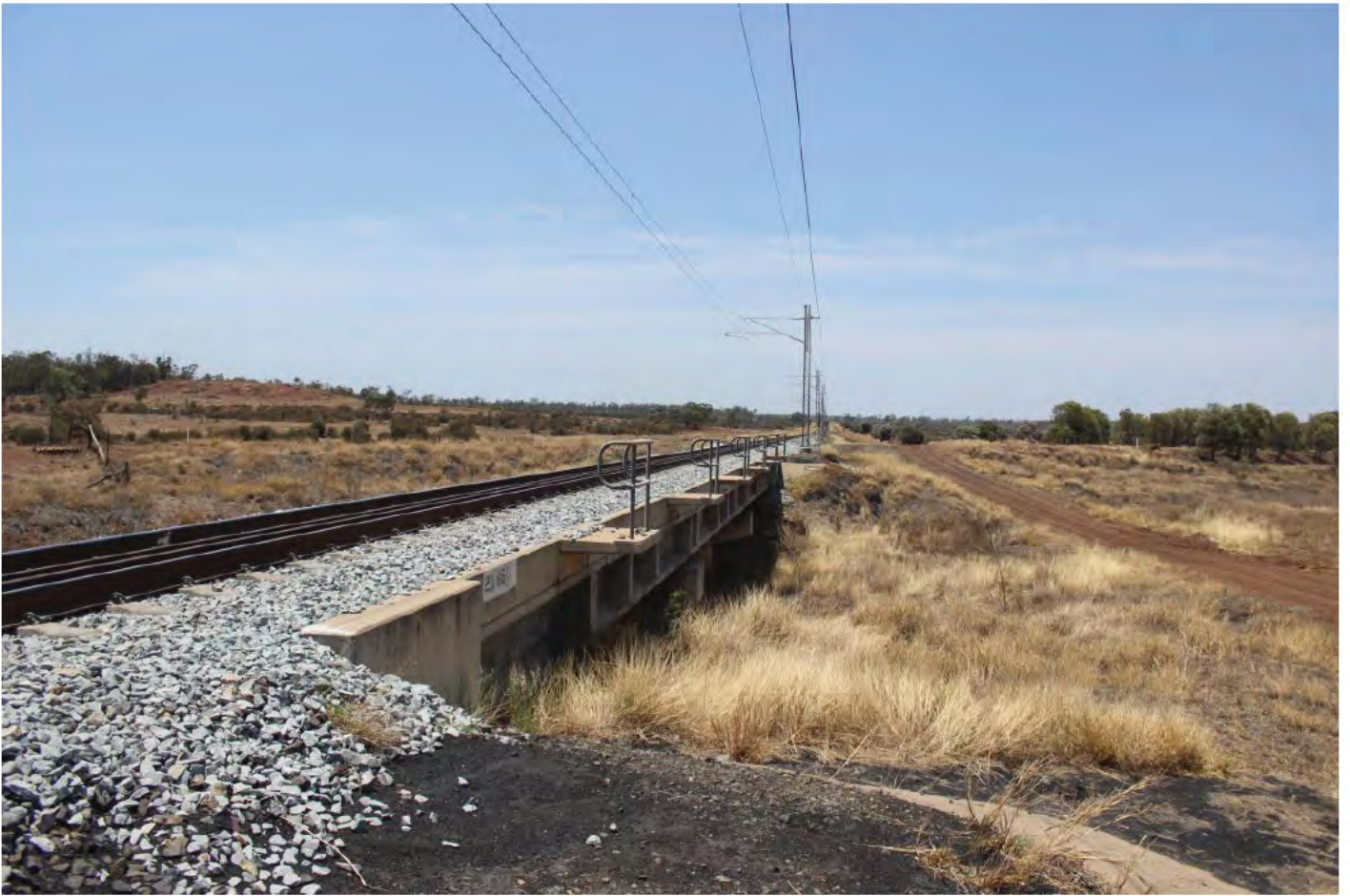
Figure 7.13: Bridge with ballast renewed in FY 19 at Wotonga on the Goonyella System
