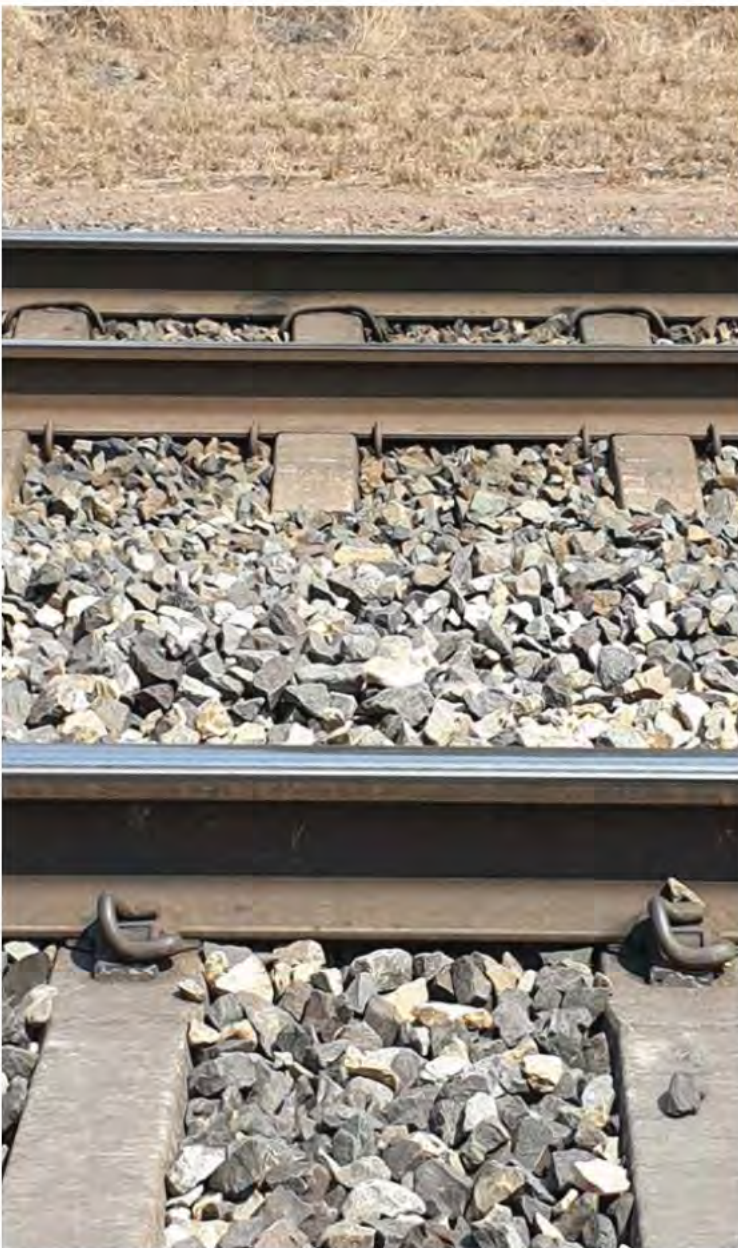
Figure 7.16: Examples of FIST fasteners on 22.5 tal concrete sleepers in the background and Pandrol e-clips on 28 tal concrete sleepers in the foreground
