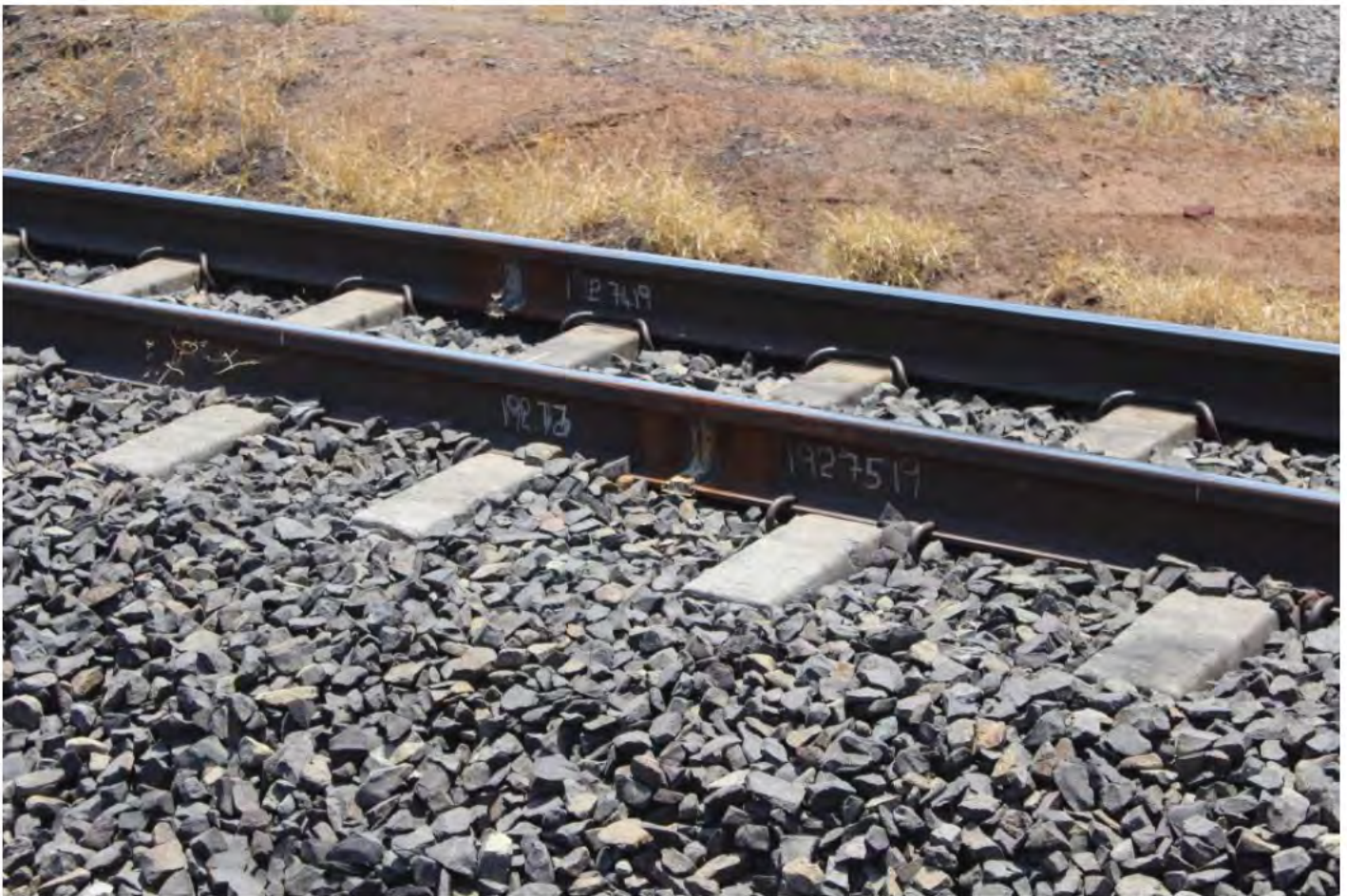
Figure 7.8: FIST sleepers on the Goonyella System
