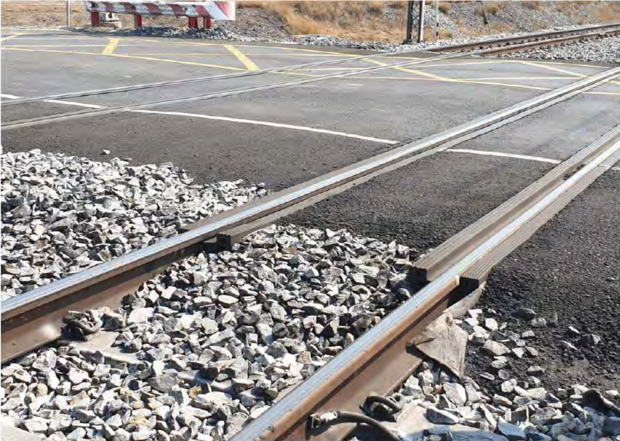
Figure 7.18: Level Crossing renewed in FY 19 scope
