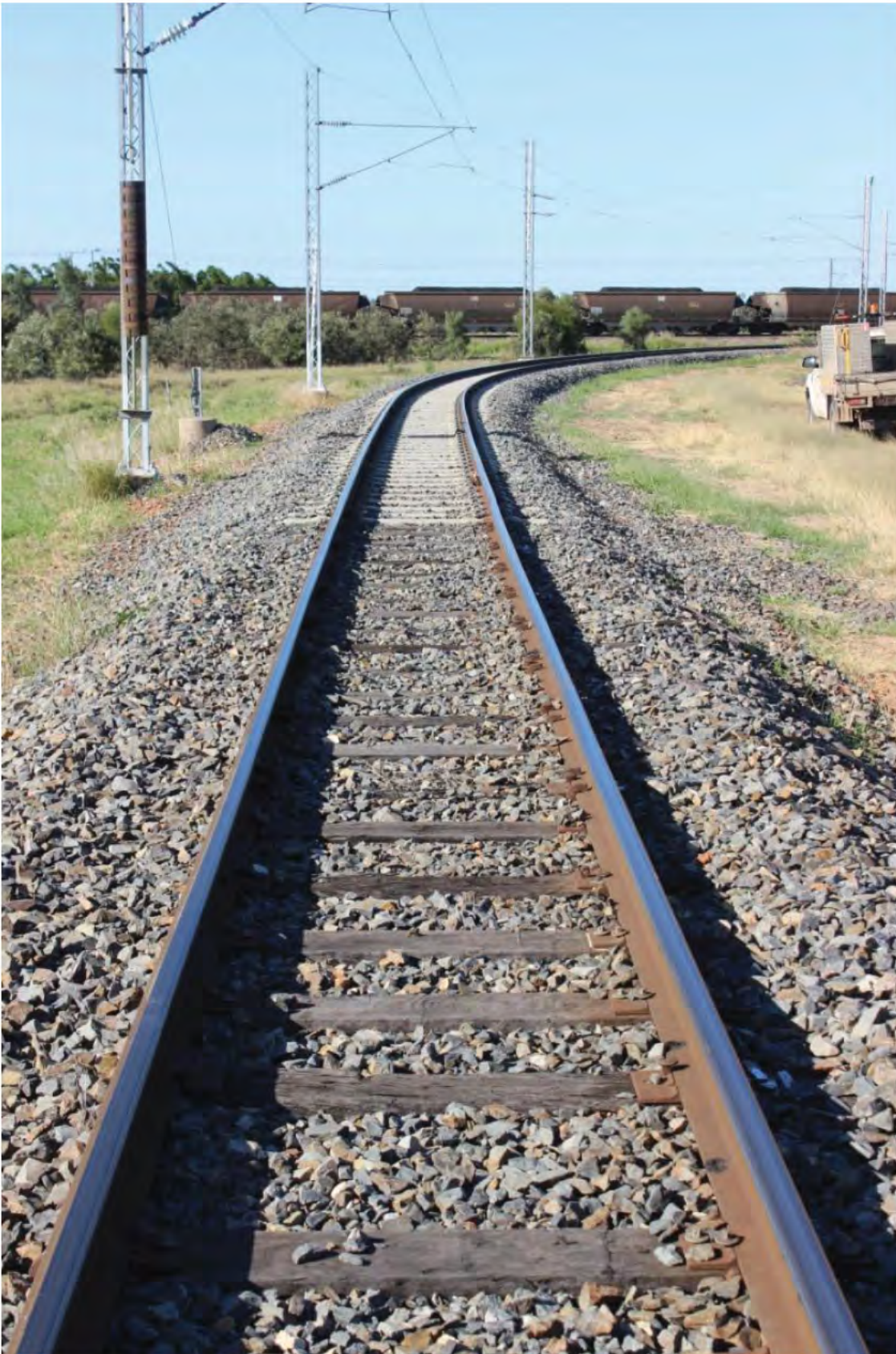
Figure 7.10: Timber sleepers and failing fasteners at Boonal Balloon Loop being replaced by concrete sleepers and Pandrol fasteners.
