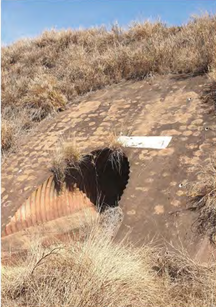
Figure 7.7: Culvert at Moranbah – Blair Athol at 27.890 km
