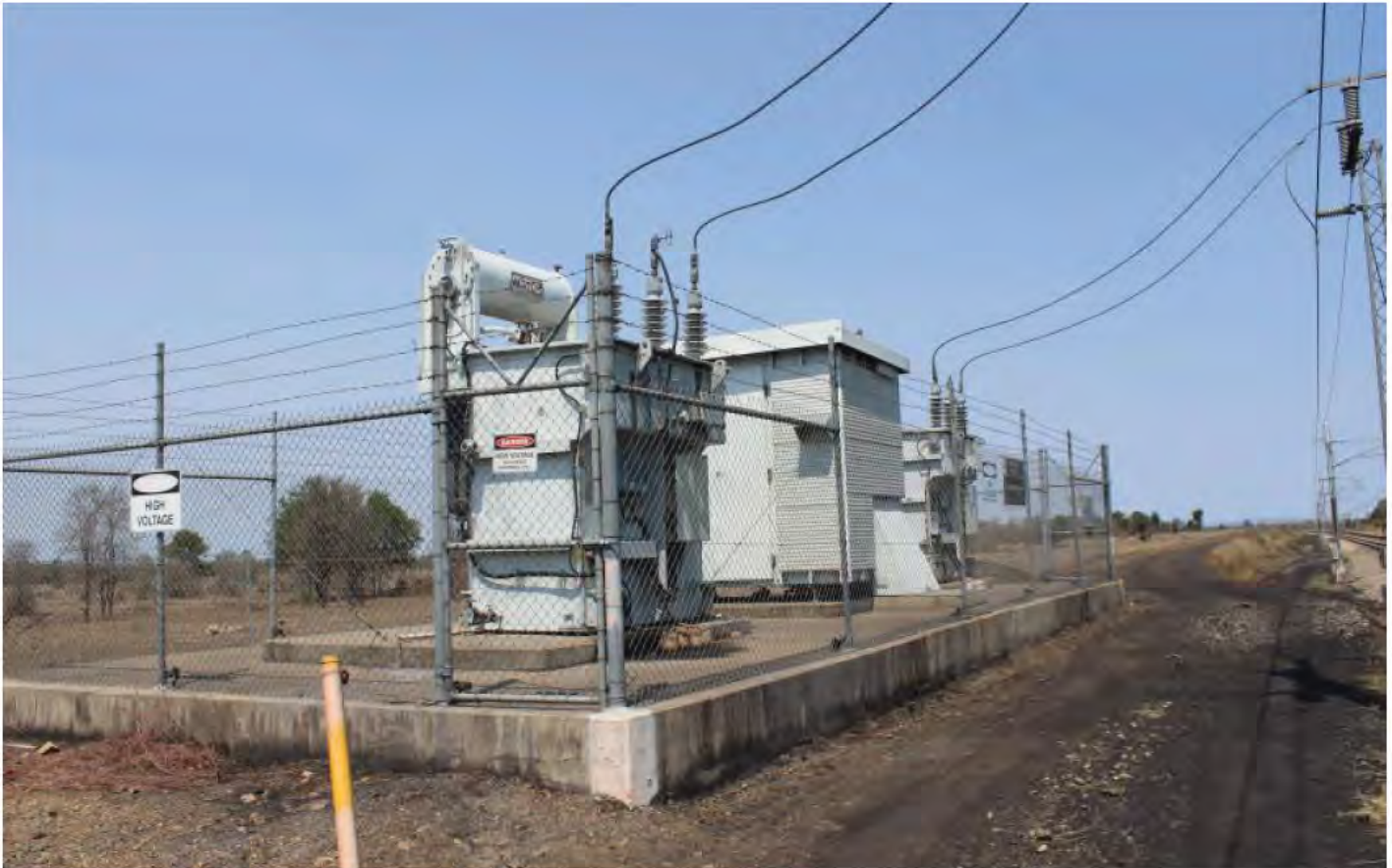
Figure 7.19: Autotransformers at 123.027 KM on the Goonyella System (Mindi to Tootoolah)
