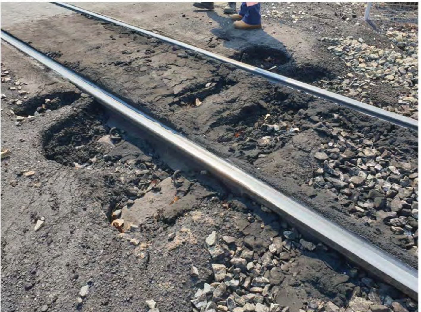
Figure 7.17: Example of bitumen damage due to ballast pumping
