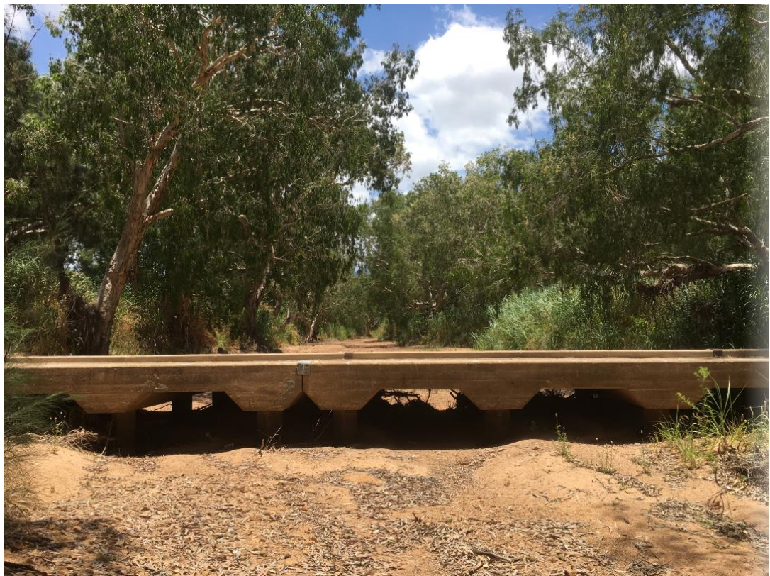
Figure 3-14 – Major Creek - Upstream Near Woodstock-Giru Road
