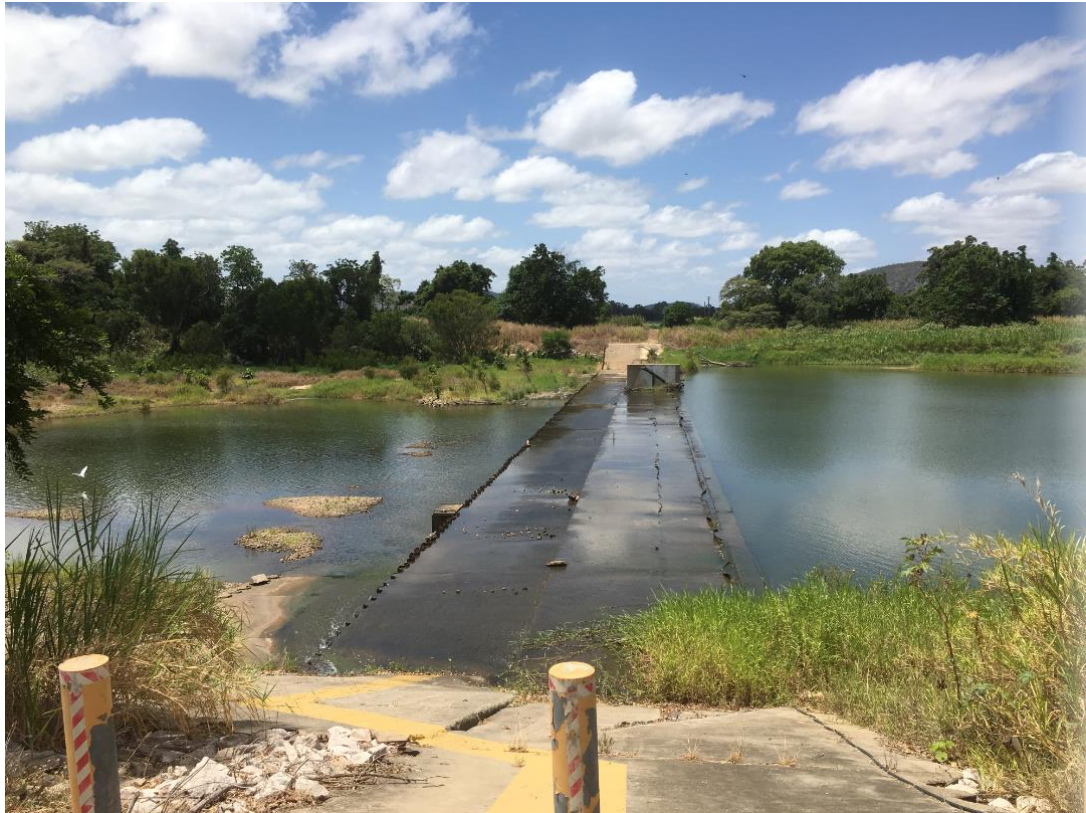
Figure 3-13 – Val Bird Weir
