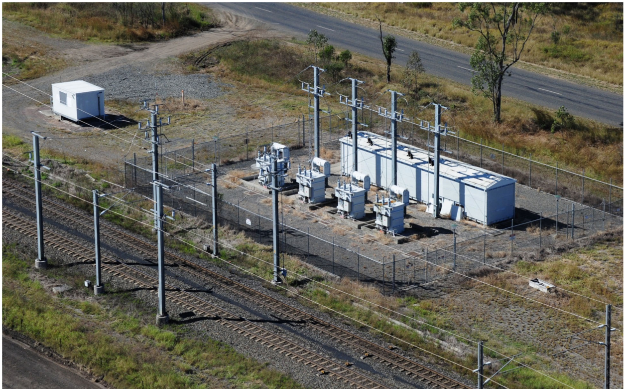
Typical Track Sectioning Cabin
