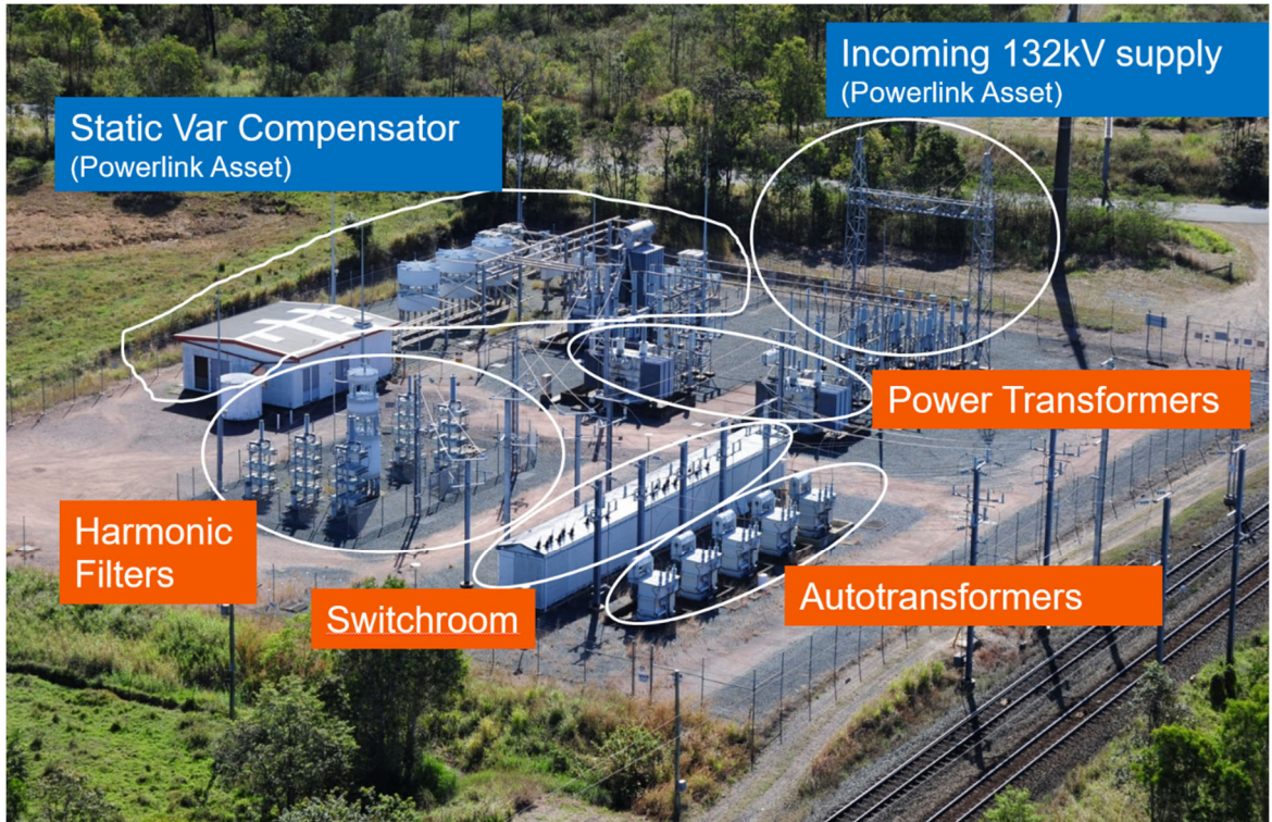
Typical Traction Feeder Station
