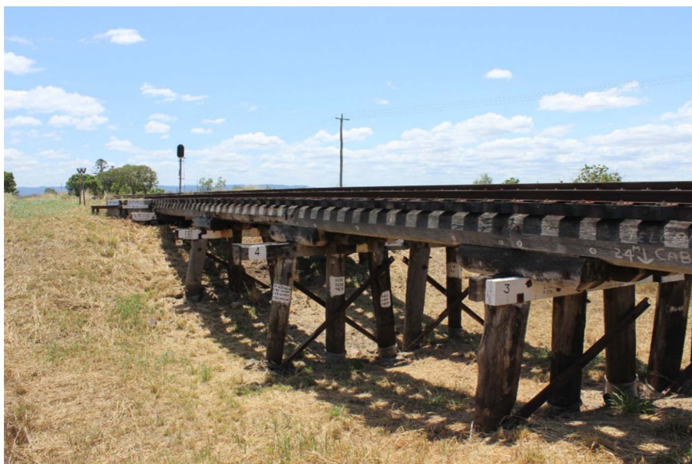
Figure 8.1: Typical West Moreton System timber at Sandy Creek
