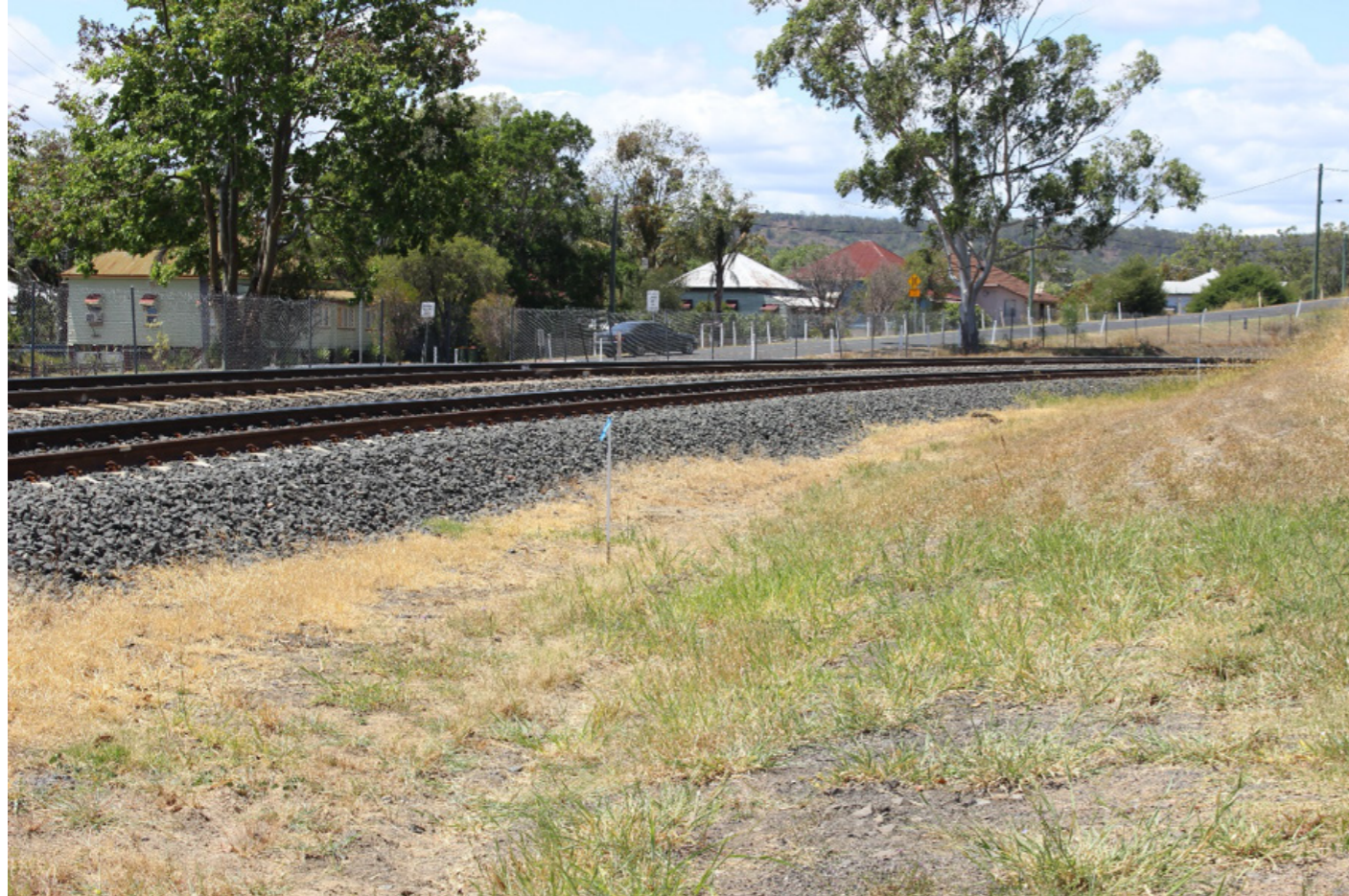
Figure 8.5: Bridge site east of Ehlma at Kilometre 135.740 on the Western Line.
