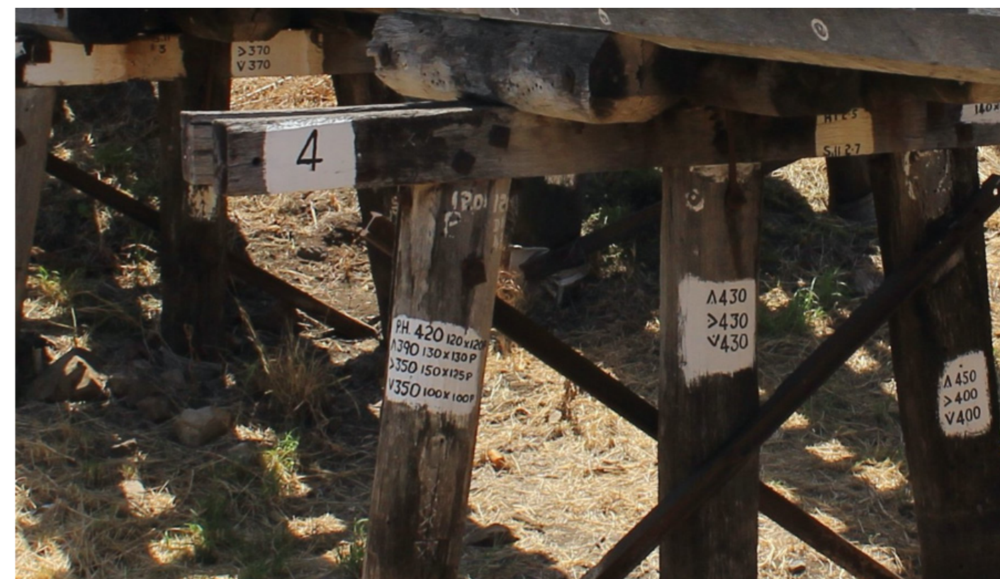
Figure 8.2: Close up of Pier 4 at Sandy Ck bridge
