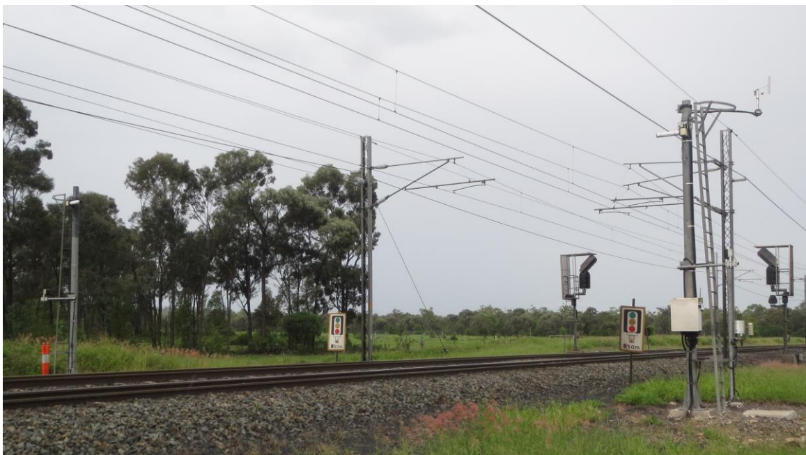
Figure 15 Coal dust detection equipment at Mindi on the Goonyella system
