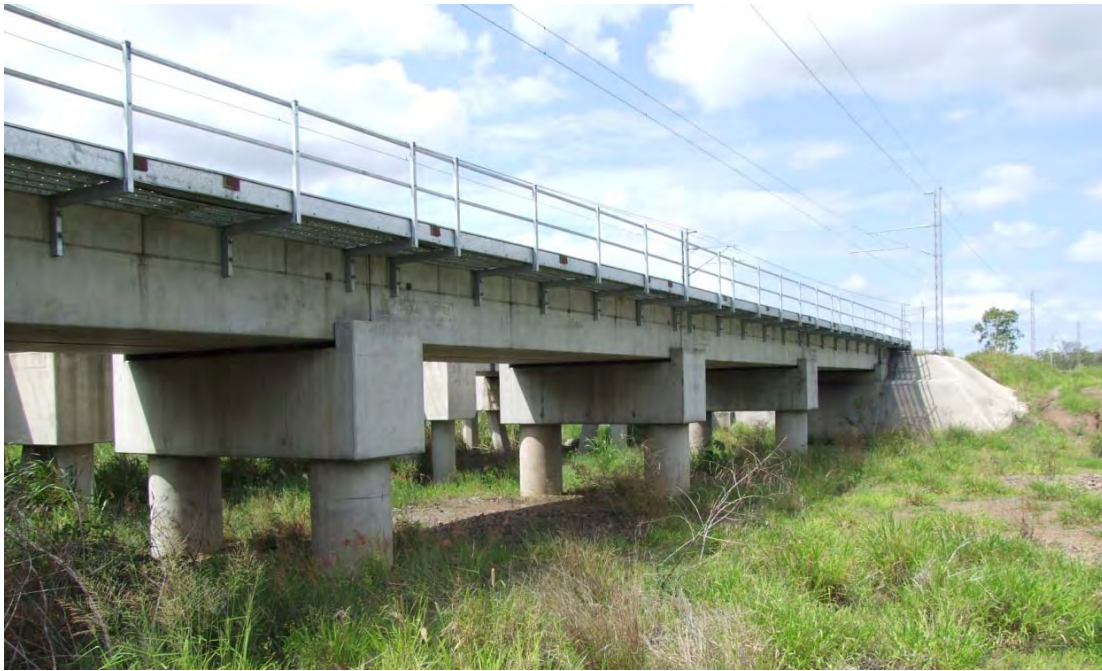
Figure 3: Bridge on the Stanwell to Wycarbah Duplication
