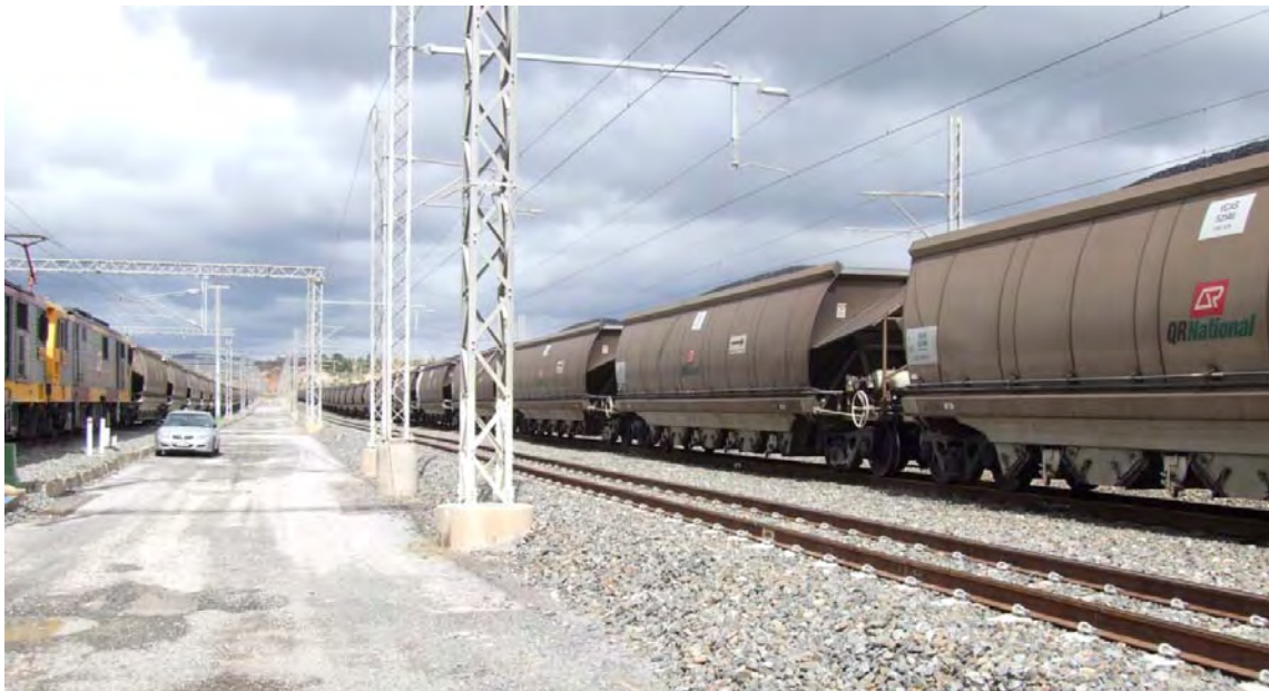
Figure 4: Callemondah 3 rd Spur
