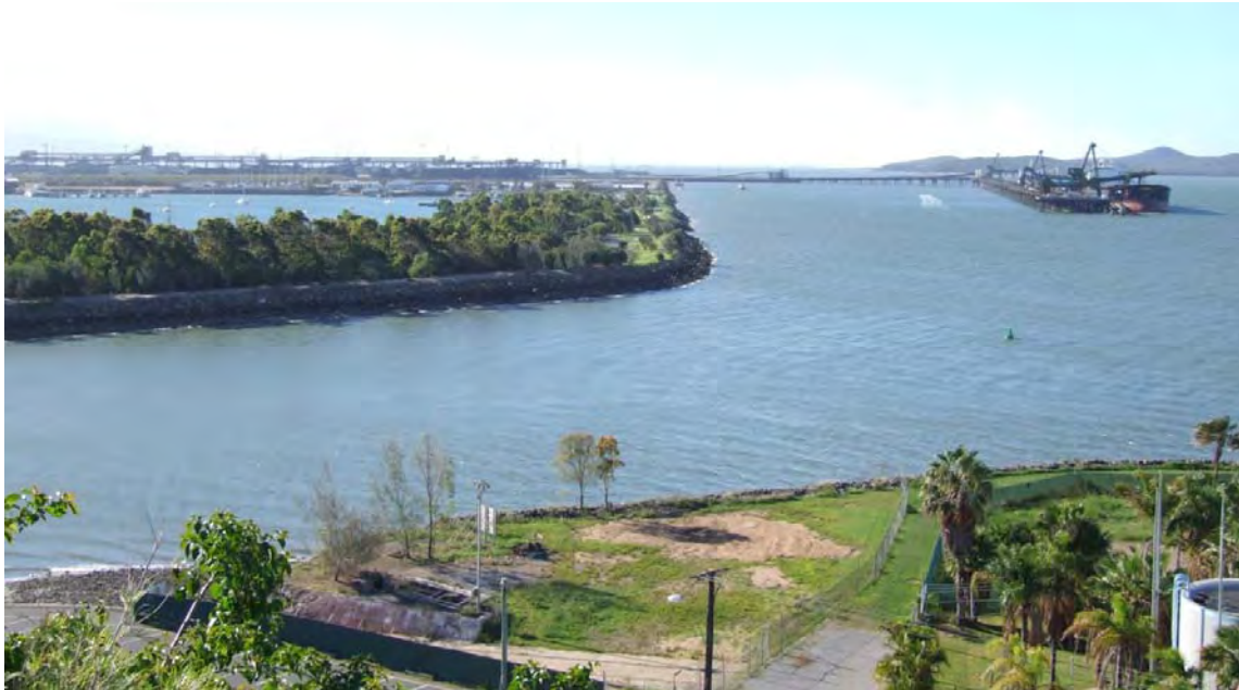
Figure 10: RG Tanna Coal Loading Facility, Gladstone
