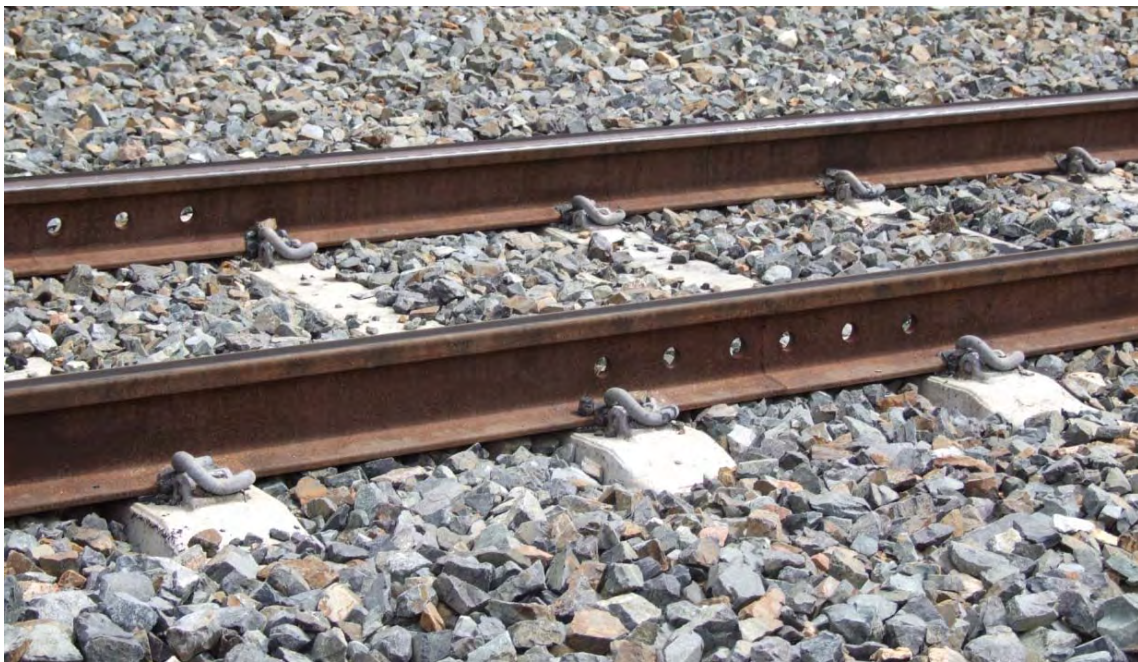
Figure 7: Reused partly worn 53 kg/m rail for the Callemondah Yard upgrade
