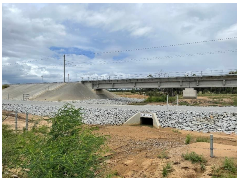
Figure 6-5 Bridge with stairs and railings and Culvert
