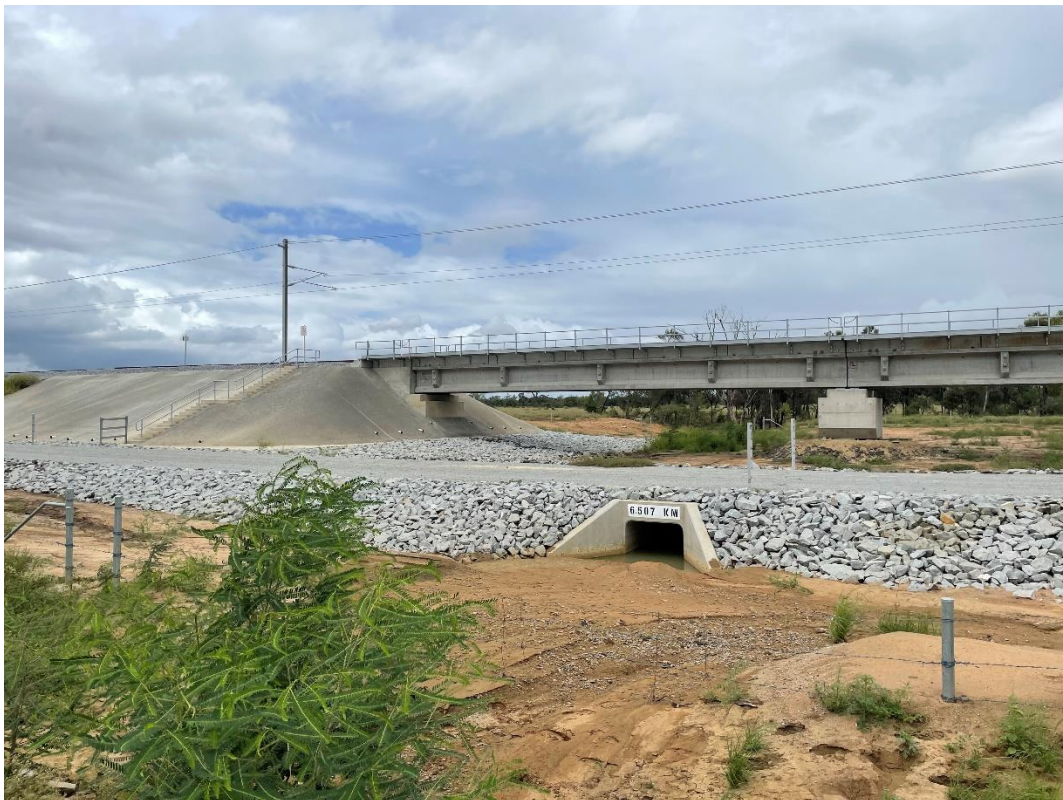
Figure 2-1 Bridge and culvert alongside the rail
