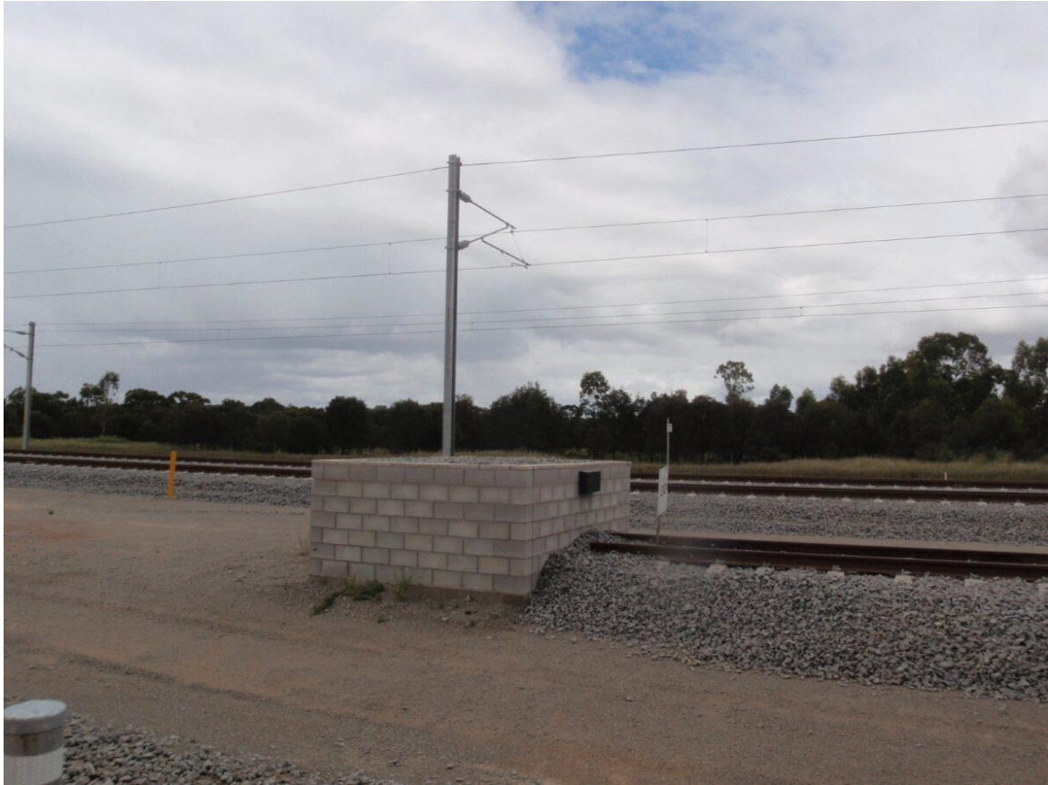
Figure 3-1 Bad order siding buff point
