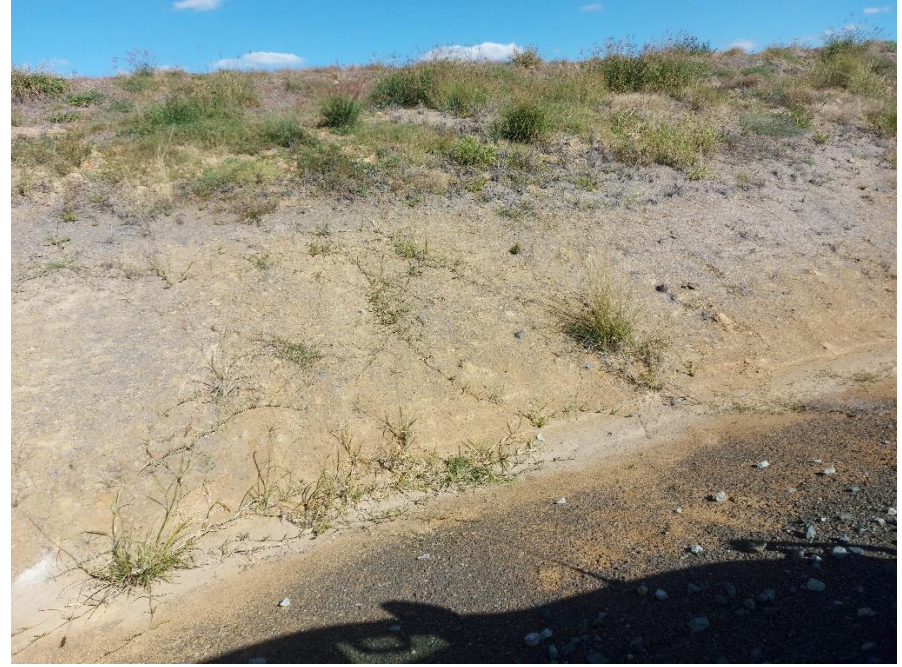
20220726_143655 – Cut and drain near CH 180.700
