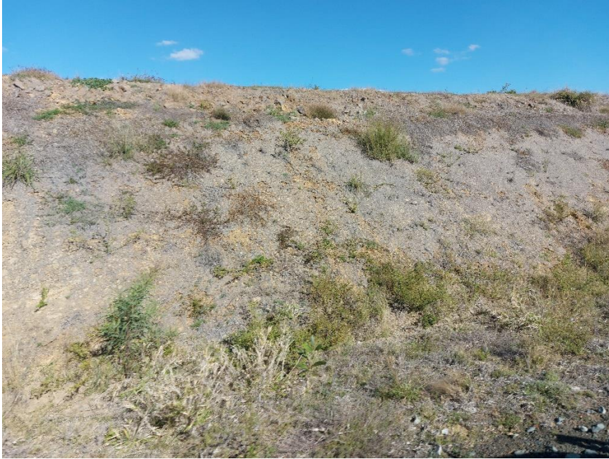
20220726_143655 – Cut and drain near CH 180.700
