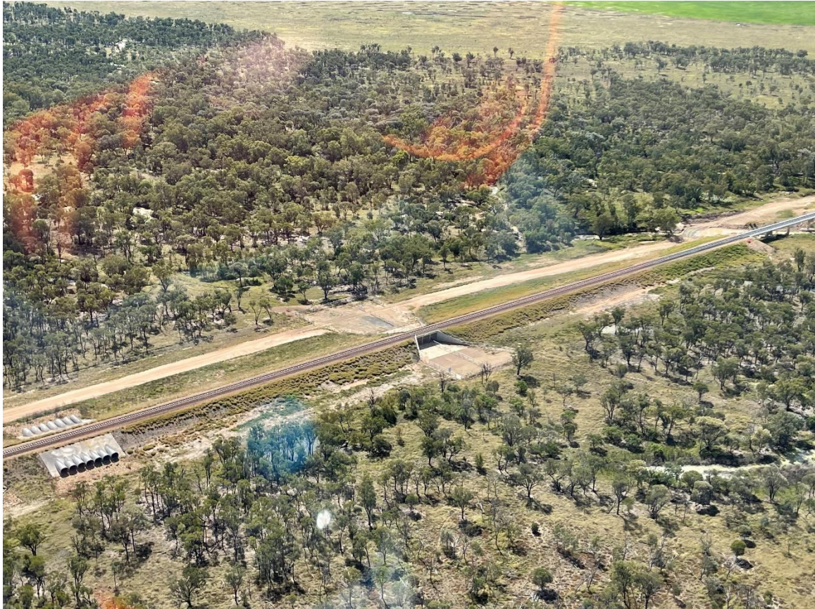
Figure 6-4 Armco culverts and structures
