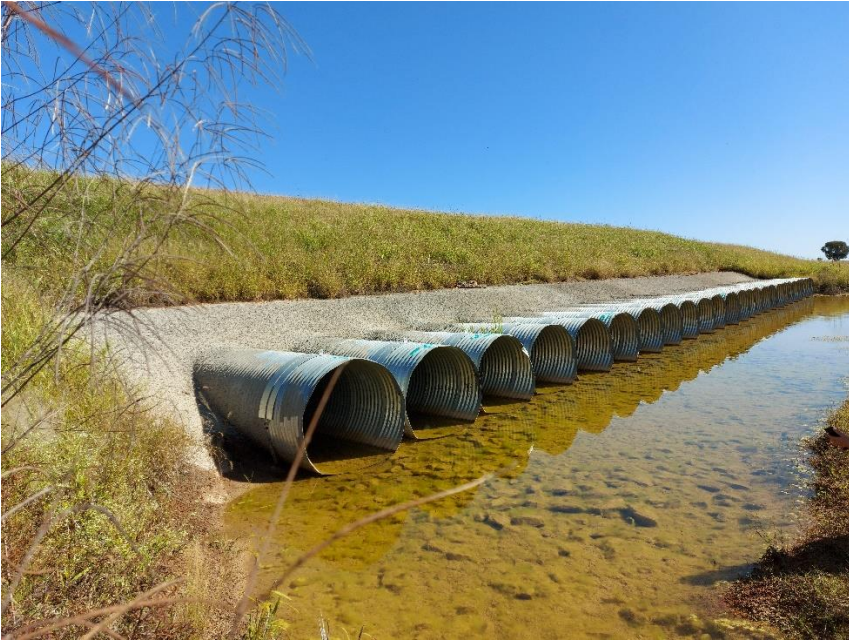
20220726_103111 – Culvert C481 at CH 382.843 - 25 x 1.2m CMP
