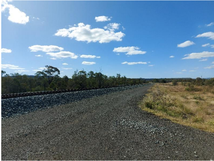
20220726_142425 – Access Road Turn around - Looking East
