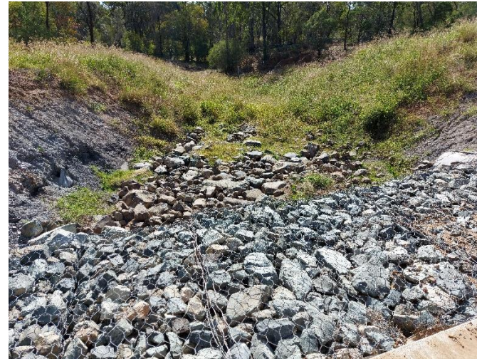
20220726_142415 – Culvert C027_2_down stream
