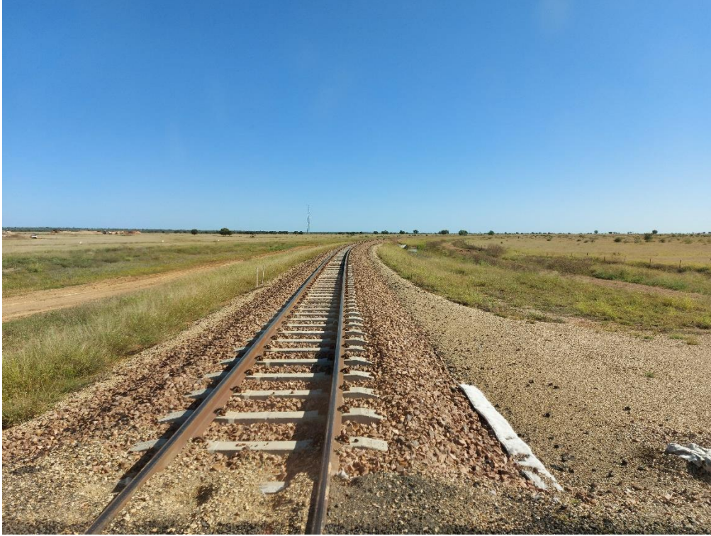
Figure 6-2 60 kg head hardened rail on concrete sleepers
