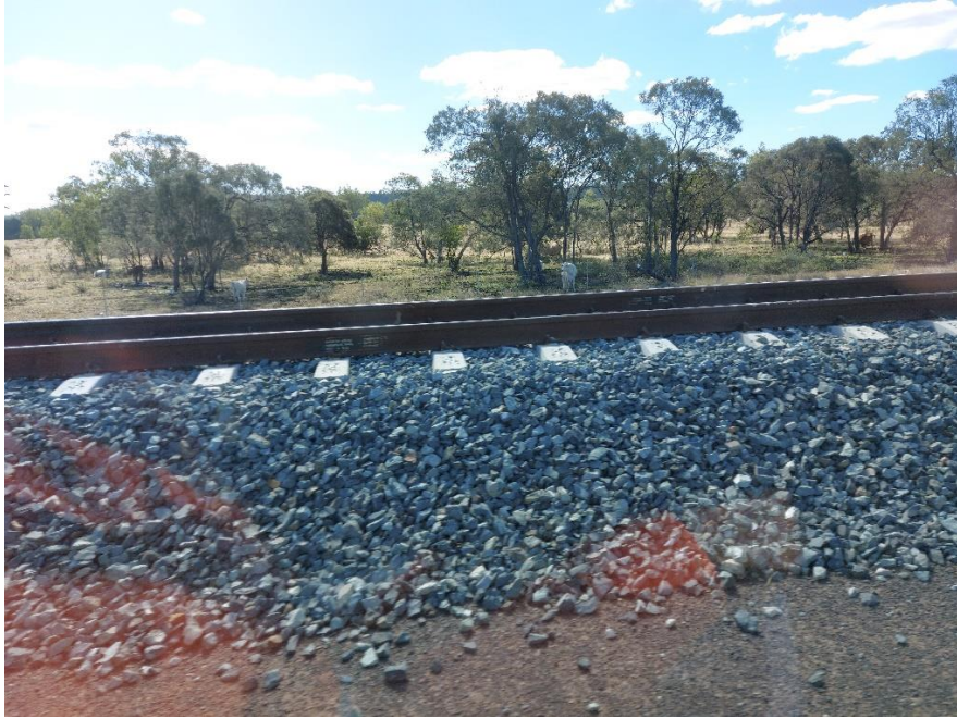
20220726_142250 – Culvert C027_3_up stream
