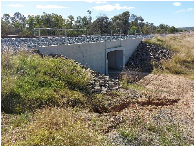
20220726_142250 – Culvert C027_3_up stream
