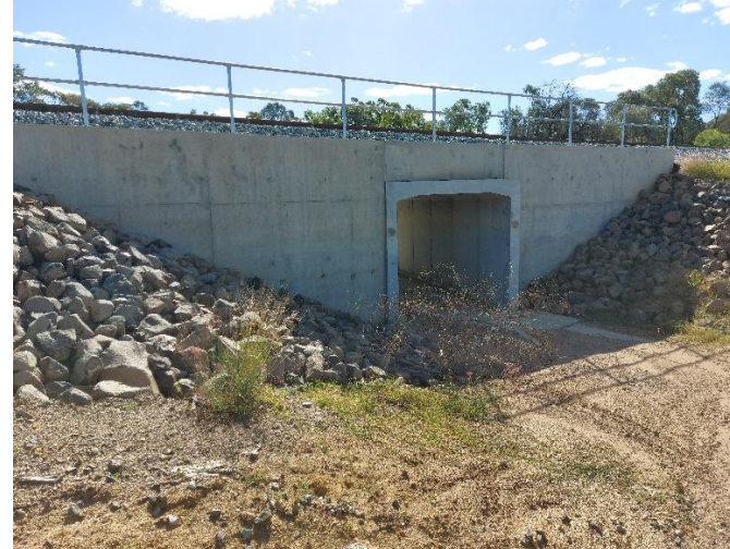
20220726_142324 – Culvert C027_4_up stream
