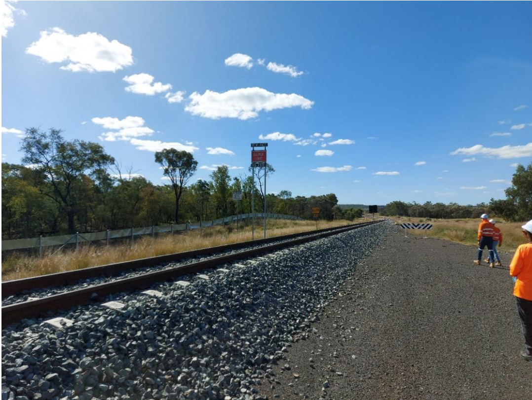
Figure 6-6 Looking East towards the connection point on Newlands line
