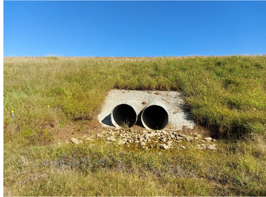
20220726_103554 – Culver C482 at CH 382.906 - 2 x 1.2m CMP
