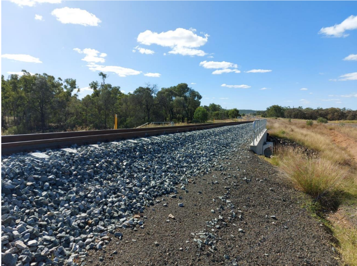
Figure 6-8 Rail was constructed in alignment with Aurizon CETS
