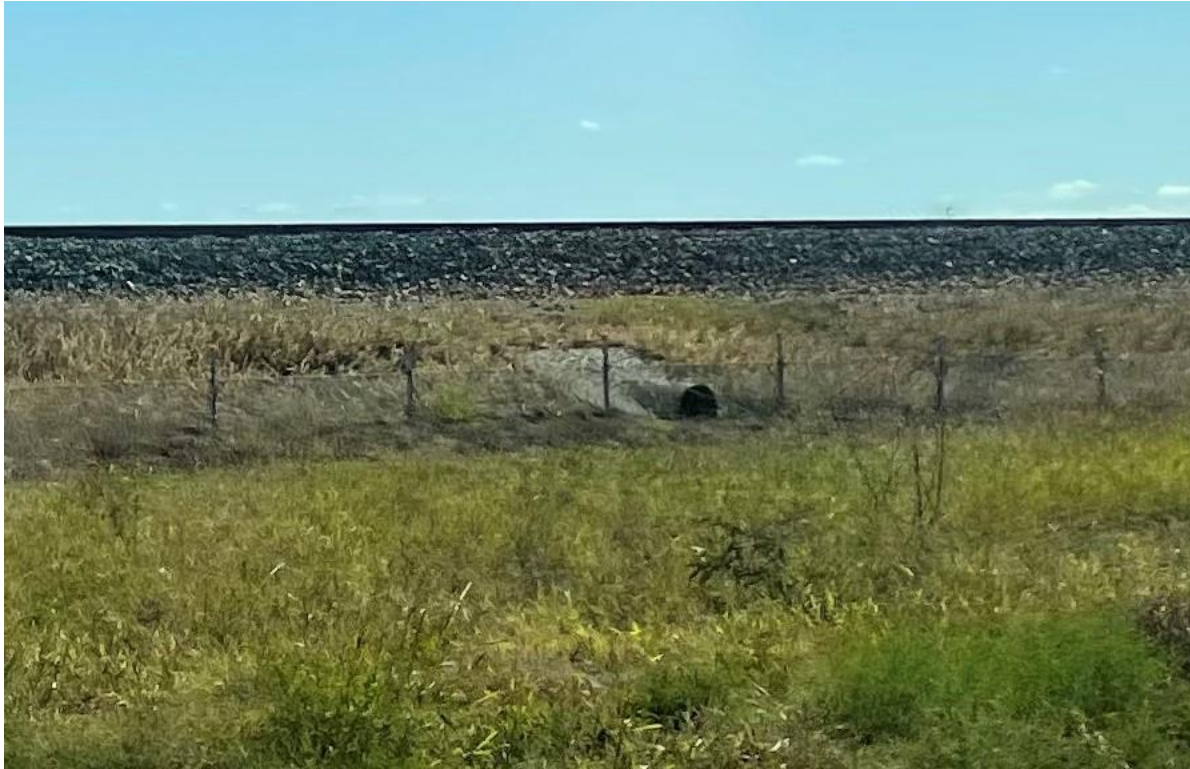
Figure 6-5 Fauna connectivity structure – snake fencing and under track tunnel (every 100m in some locations)
