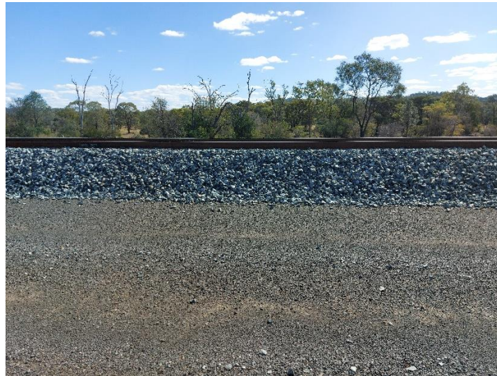
20220726_141436 – Track structure near Km 181
