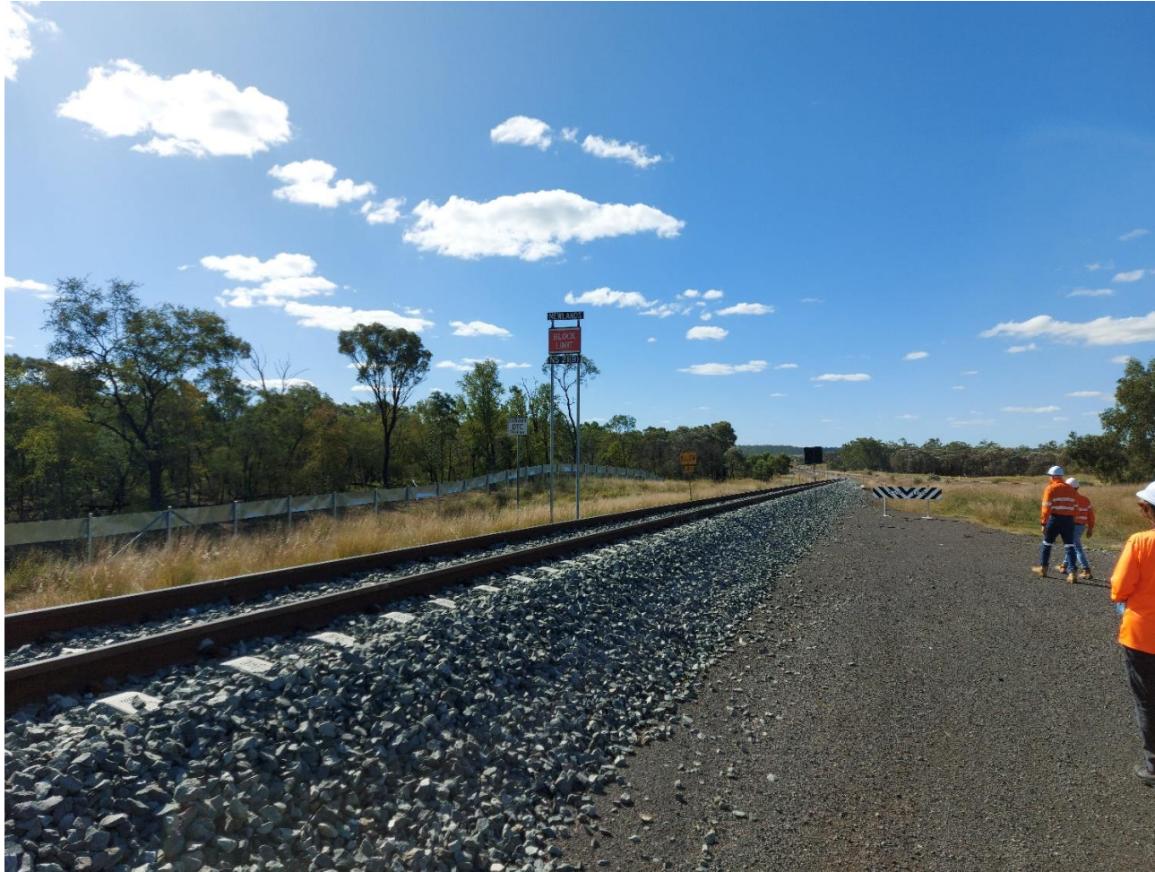
20220726_142009 – Looking East towards the connection point on Newlands line
