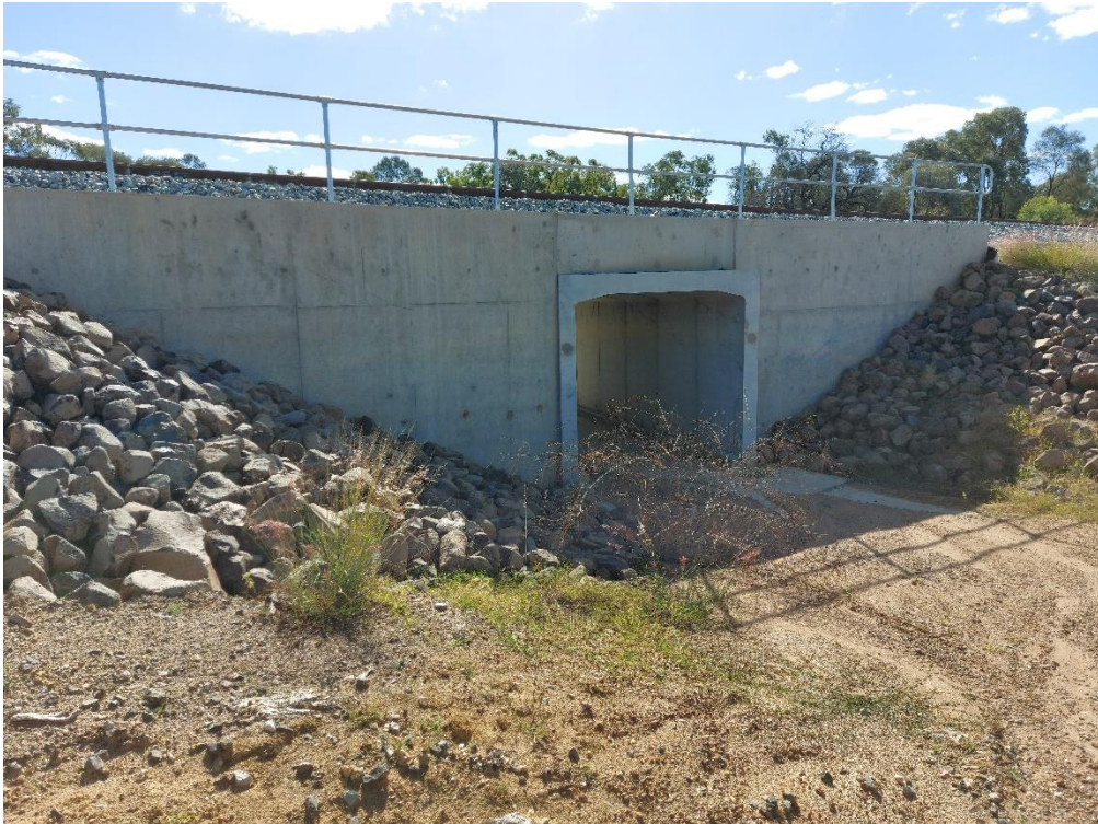
Figure 6-3 Reinforced concrete culvert
