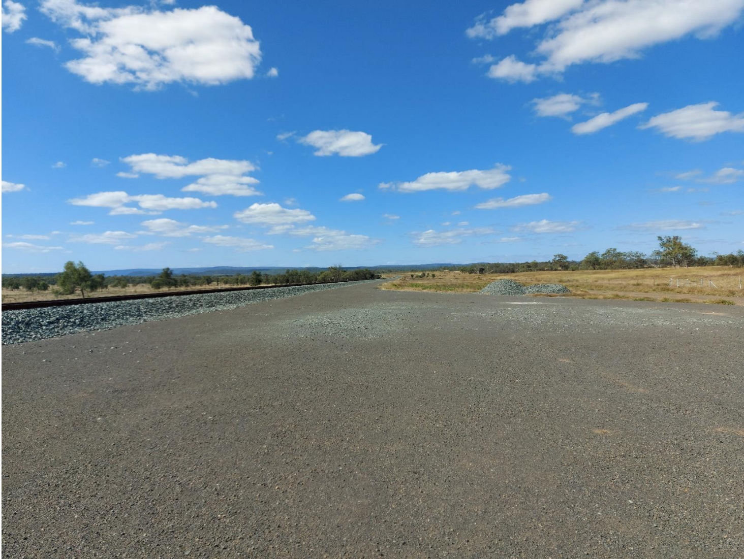
20220726_135551 – Formation widening/access pad Rail In- Looking East
