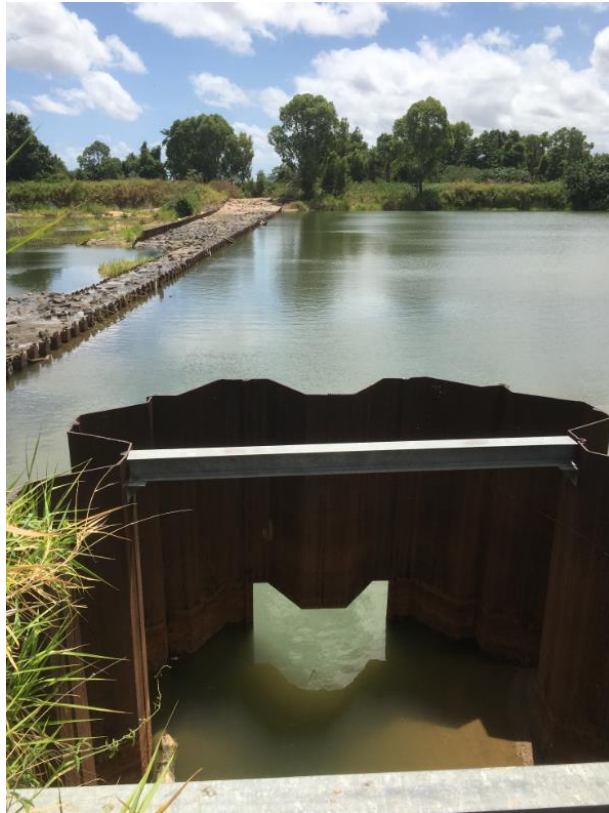
Figure 3-11 – Giru Weir – Intake to Bypass Pipe
