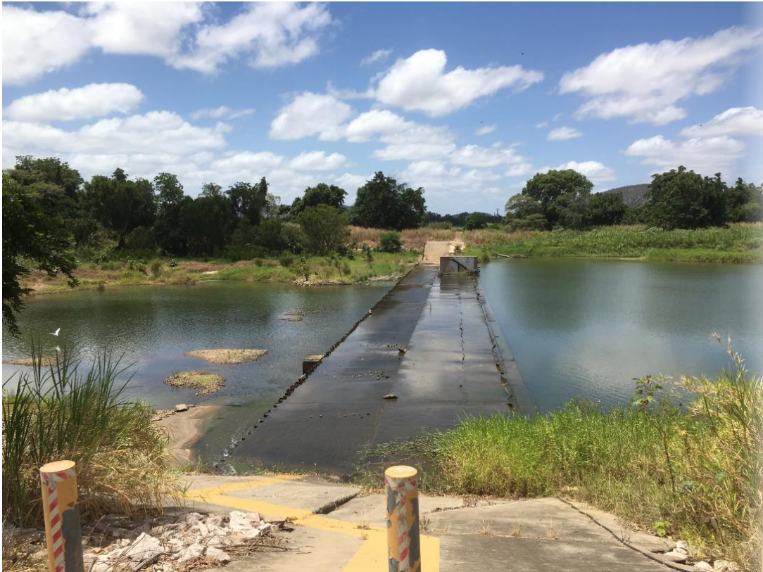
Figure 3-13 – Val Bird Weir
