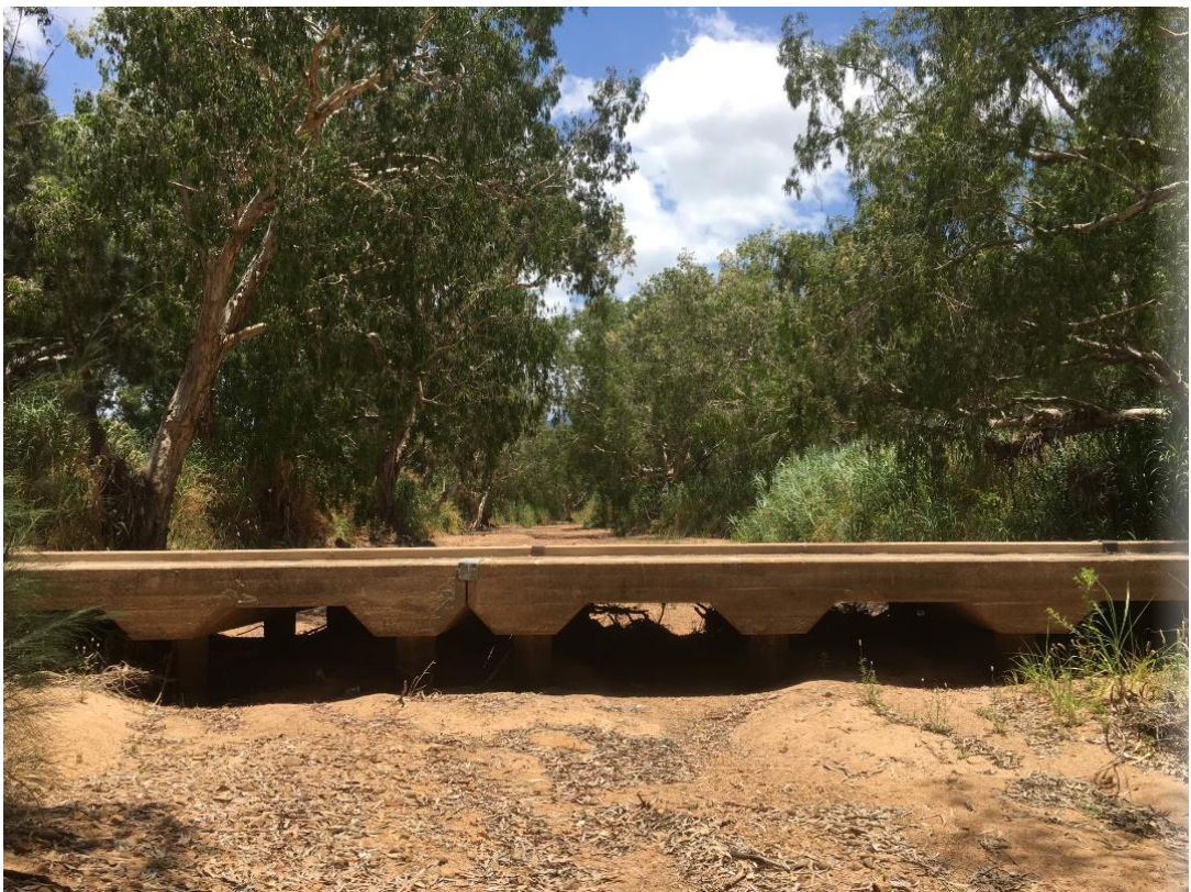
Figure 3-14 – Major Creek - Upstream Near Woodstock-Giru Road
