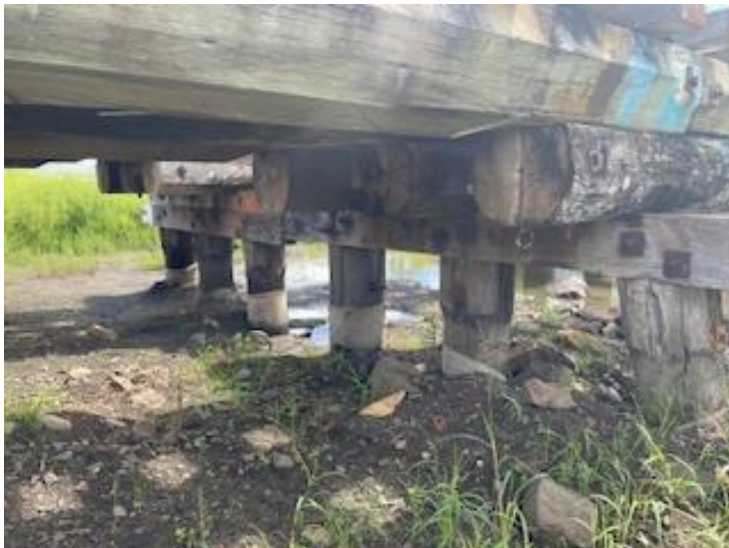
Figure 5-2 WMS timber bridge
