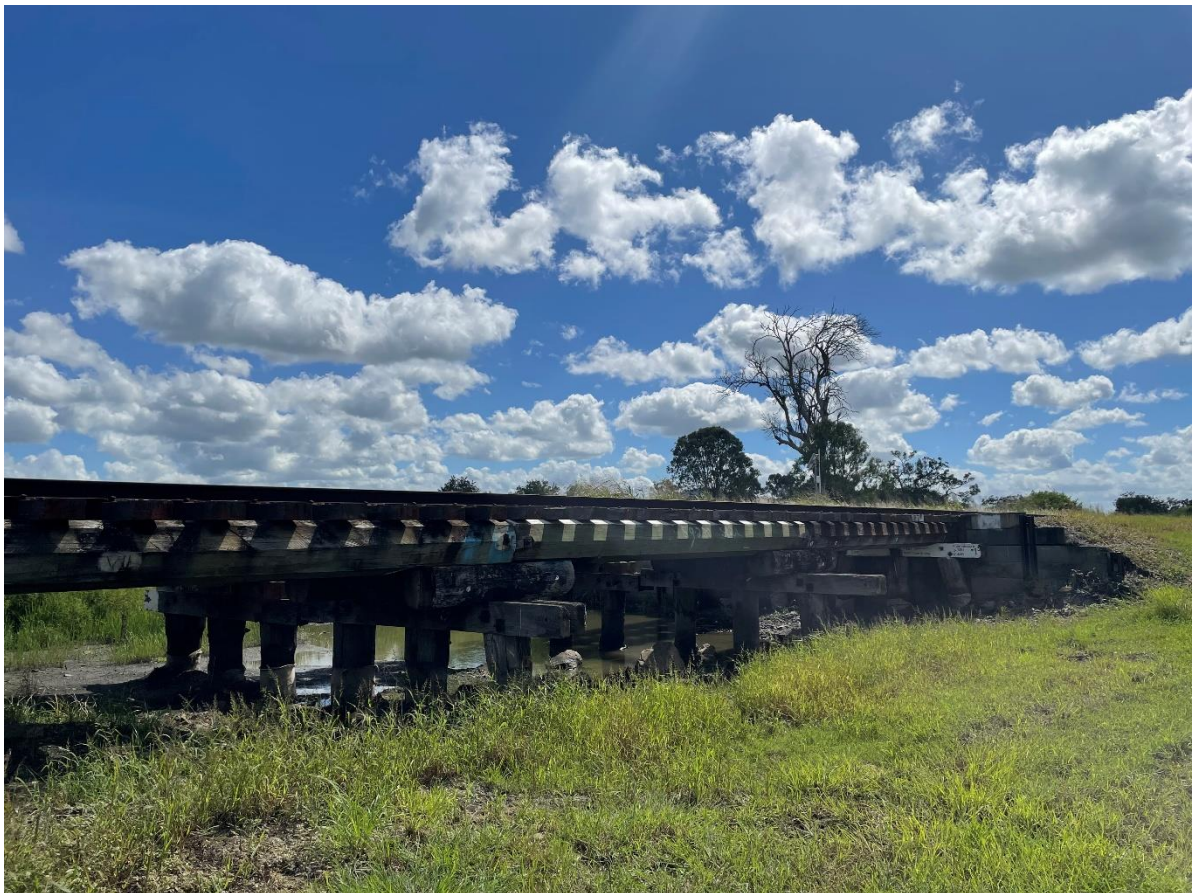
Figure 6-1 WMS Track and Bridge
